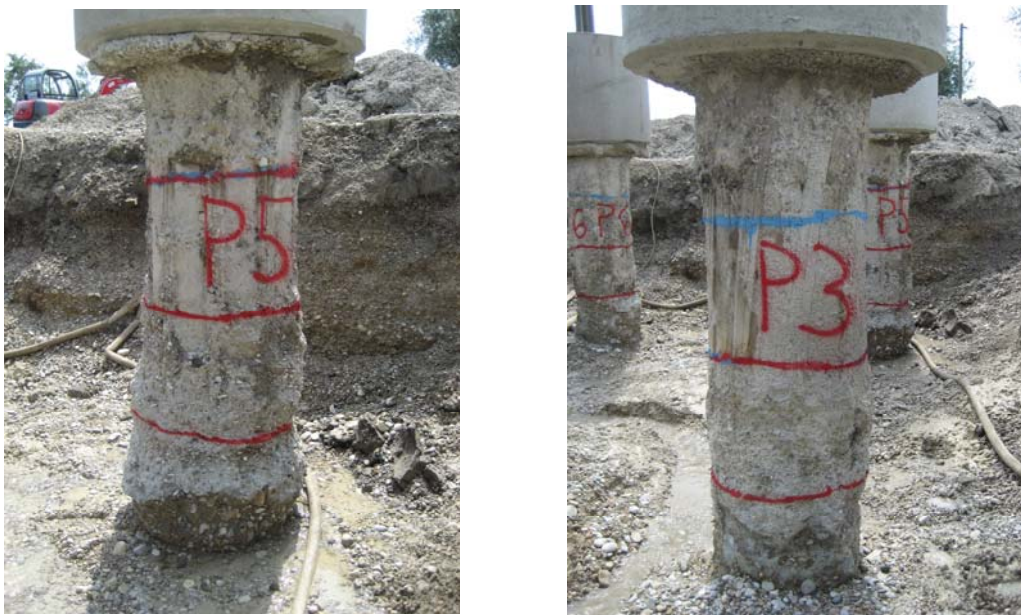
Figure 4.4: Photos of pile P 3 (bentonite) and pile P 5 (polymer)
