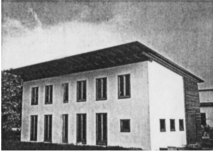
Figure 9. External View of the Passive House (Kleiner (ed.), 1995:82-83)
