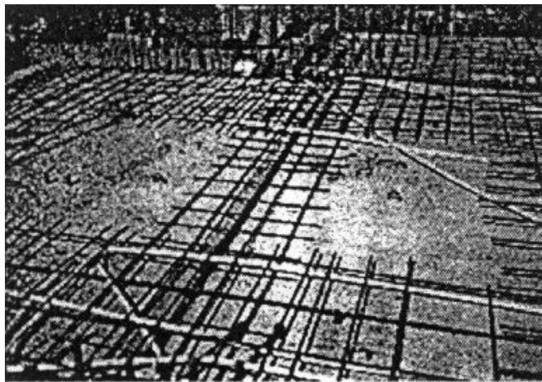
• Figure 17 - Semi-precast slab construction
