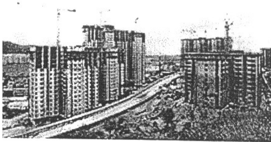
• Figure 13 - Typical public housing construction sites in Hong Kong
