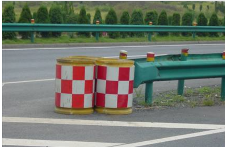
Figure 6. Crash Cushions in an Interchange Gore Area
