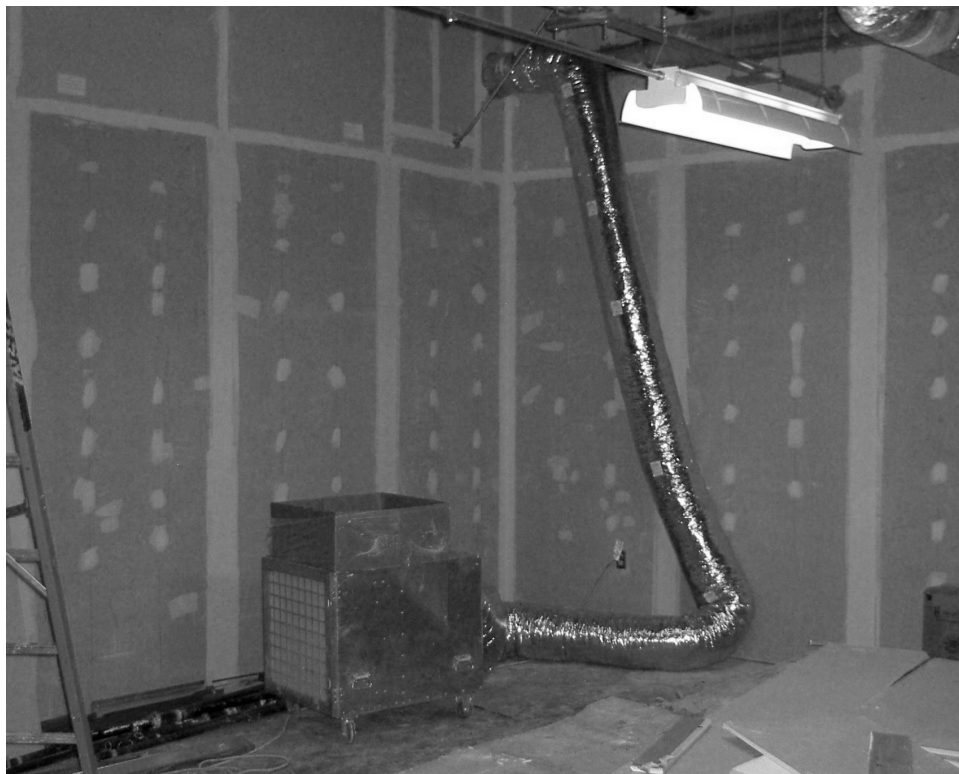
Figure 2 – Negative Air Pressure HEPA Filter
