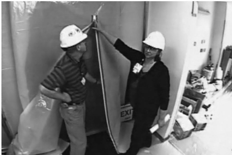
Figure 4 – Dust Barrier at Door
