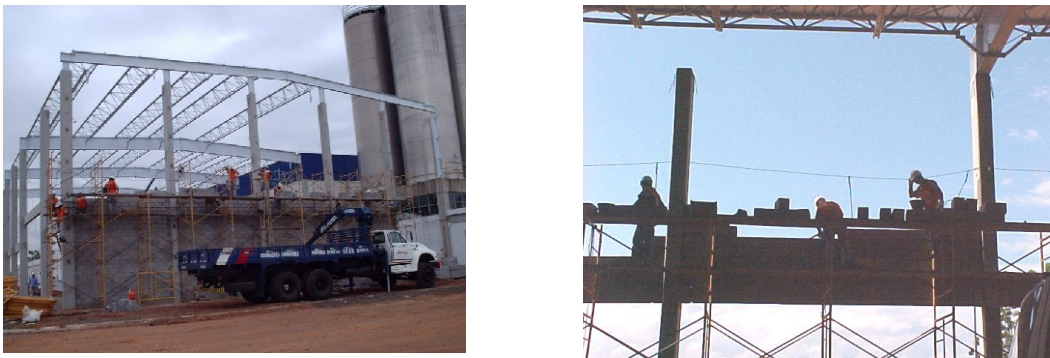
Figure 1. On the left: steel framing and pre-cast framing. On the right: pre-cast columns in which holes were made to allow the passage of lifelines.
