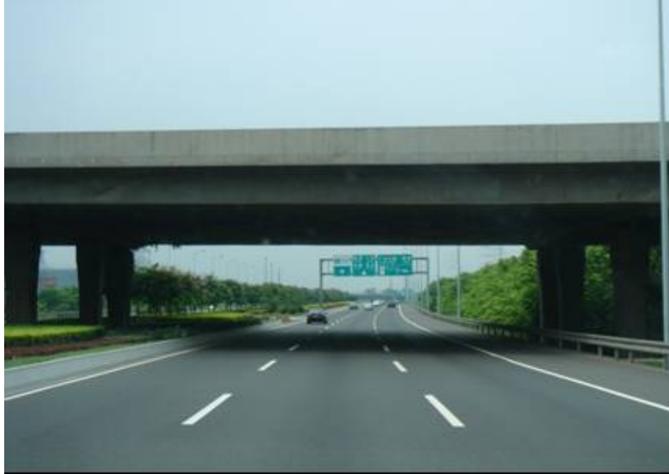
Figure 9. Curbs under an Interchange Bridge
