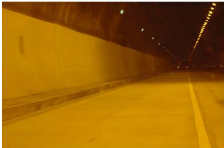
Figure 5. Only Some Lights Are on in the Tunnel
