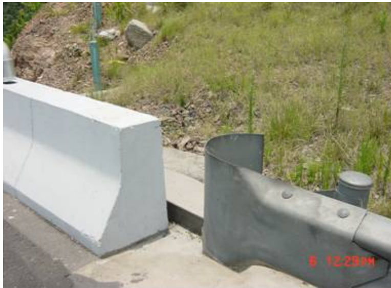
Figure 2. Space between Bridge Rail and Guardrail
