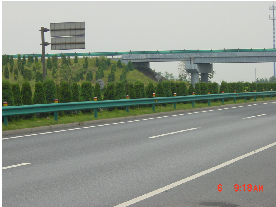
Figure 8. Curbs and Guardrails in the Median
