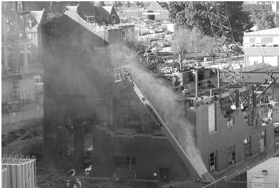
Figure 1 – Water Droplet Dust Control
