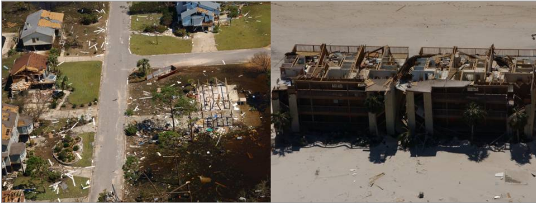
Fig 1. Debris and damage to residential and commercial structures during Hurricane Ivan, Pensacola Beach, Florida, 2004 (Grosskopf, 2004).
