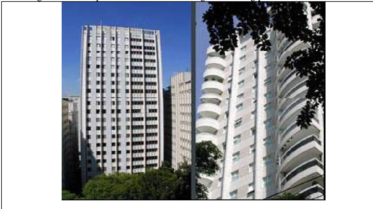
Figure 3 - Façade before and after the renovation process (photo from PROJETO DESIGN, ed. 286, Premio Asbea 2003, p. A47)
