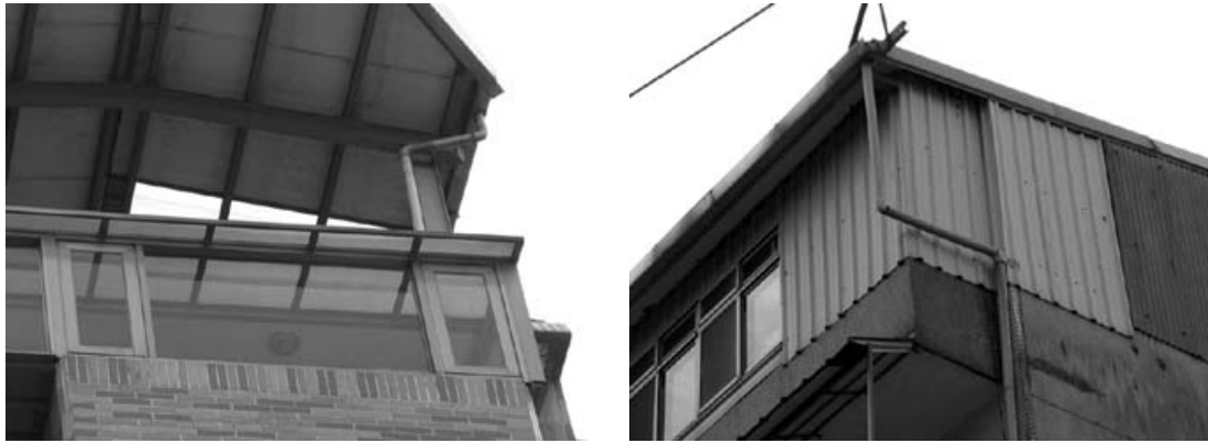
Figure 9. Reinforce concrete structure building with additional steel roof frame
