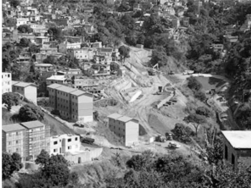
Figure 1.1 Urbel's buildings are usually set in artificial plateaus in favelas revealing that the steep topography and geomorphology of each site are underestimated. The wide streets are designed as they are in the formal city. Photo credit: Urbel .
