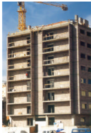
Single leaf wall in lightweight concrete
