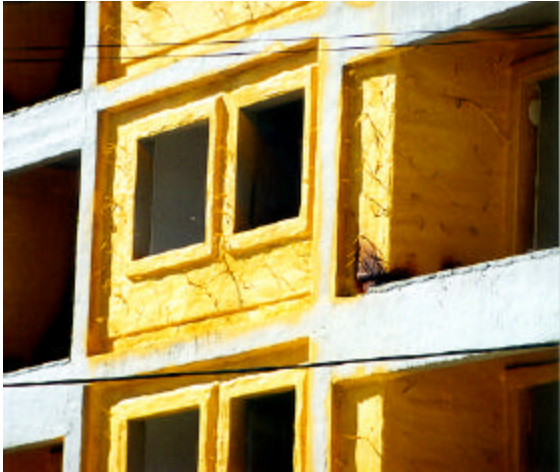
a) projected polyurethane foam
