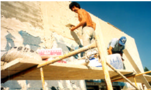
Single leaf wall in lightweight concrete
