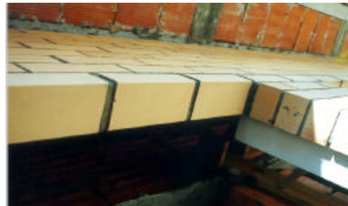
Single leaf wall in lightweight concrete
