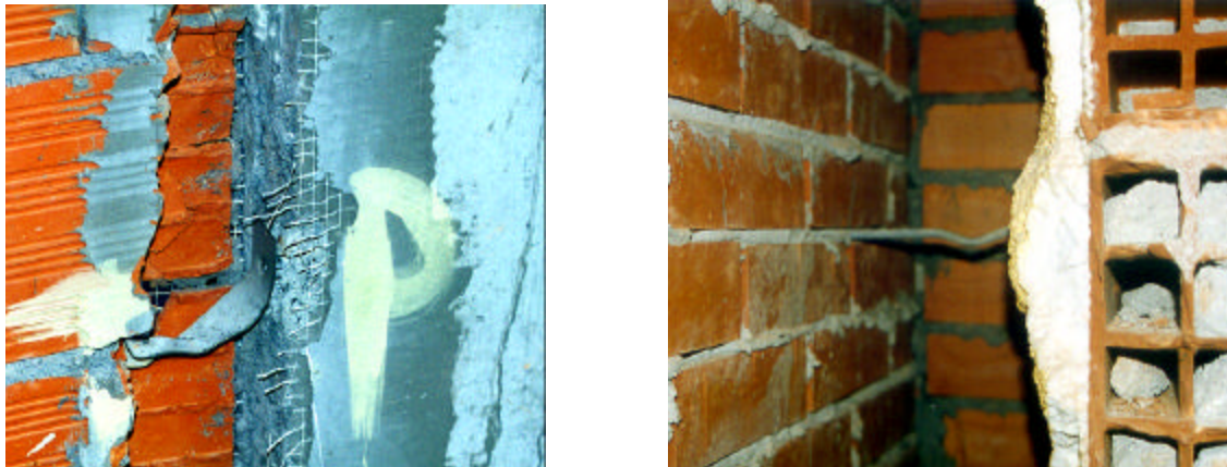
Figure 5: Examples of some ties and connectors used in Portugal
