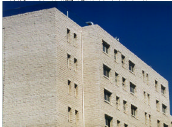
c) Split dense aggregate concrete units
