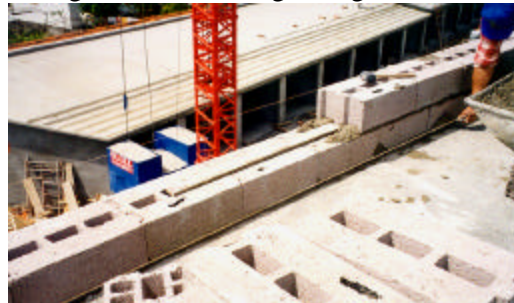
Single leaf wall in lightweight concrete
