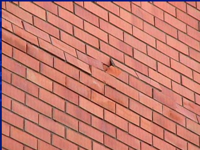
Expansion of bricks
