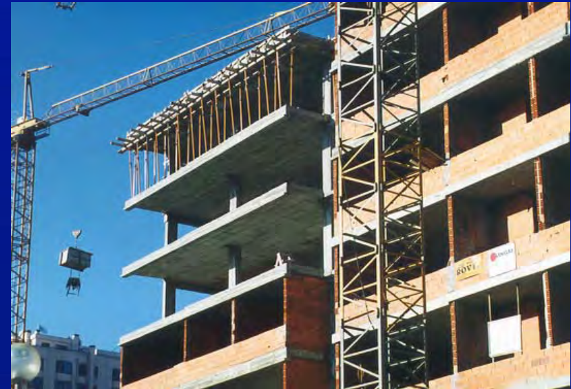
Excessively deformable slabs
