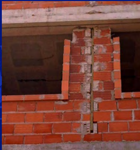
Deficient interaction with the structure
