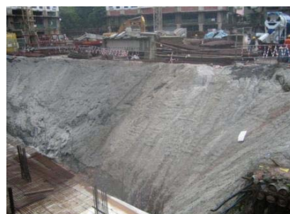
Fig. 8 Paving Up of Slope with Concrete
