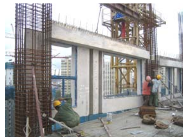
Fig. 13 Cast-in Windows to Precast Facade
