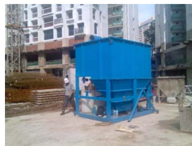
Fig. 9 Silt Water Treatment Tank
