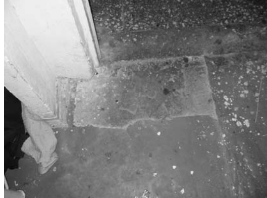
b. Degradation of the linoleum floors
