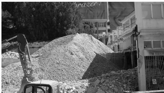
Figure 4. Concrete, masonry and ceramic materials after demolition and size reduction, at Estoril-Sol working site
