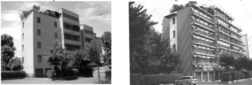
Figure 1-2: Ventiladed façade in the refurbishment of a residential building in Modena (before-after)
