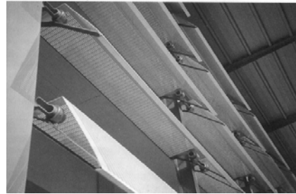
Figure 5-6: Overlapping of lamellas and panels solar shadings in the refurbishment of an office building in Lecce
