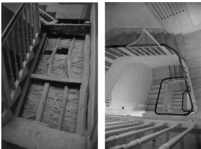
Figure 5. Staircase: (a) during deconstruction process and (b) after renewal.
