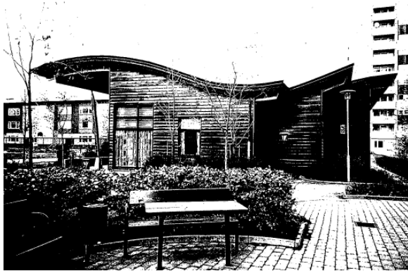
Figure 7. A multi-functional common house for the housing area Norra Lövgärdet, Gothenburg, created by using the basement and the first floor of one of the central buildings which was dismantled. The concrete construction of the original building was used as far as possible. The new building is announcing its specific nature by partly glazed façades and a spectacular “green” roof.
