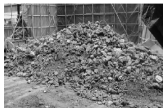
Figure 1. Sorted broken concrete and steel stockpiled separately (Guidelines for selective demolition).
