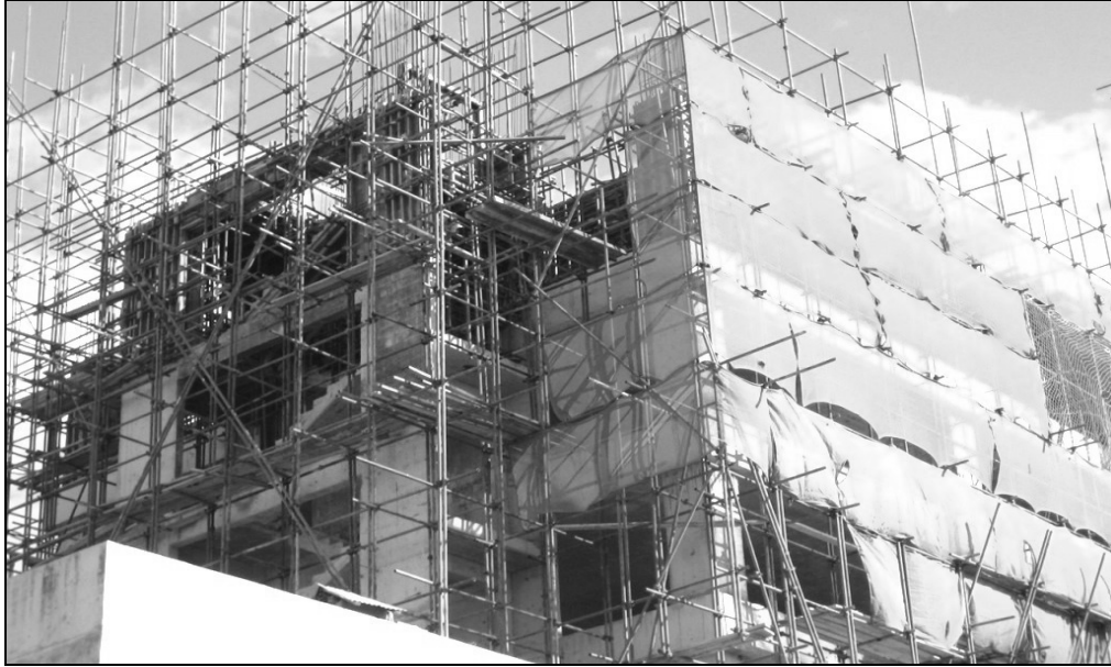
Figure 1. One of the six sites (Table 1) where both wood and steel were used for temporary formwork and scaffolds in casting in-situ reinforced concrete in the construction of multi-storey buildings in Dar es Salaam City, Tanzania (field observation)
