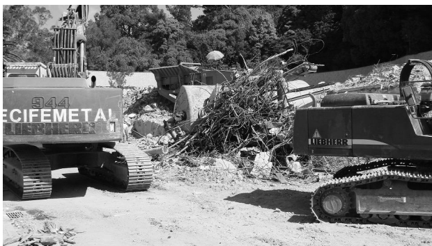
Figure 5. Reinforcement steel and other metals separated for recycling, at Estoril-Sol working site
