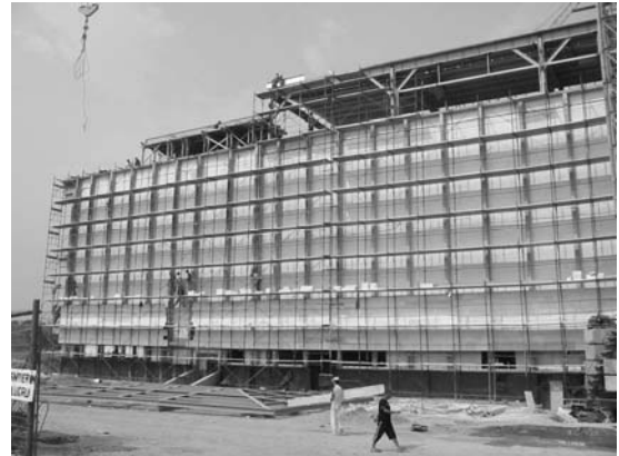
a. Detail from the installation of the envelope walls on the Southern facade b. General view of the Southern facade
