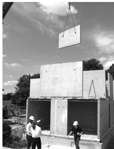
Figure 6. Mounting of the building carcass.
