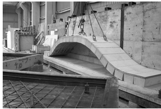
Figure 7b: Arch Unit during Lifting
