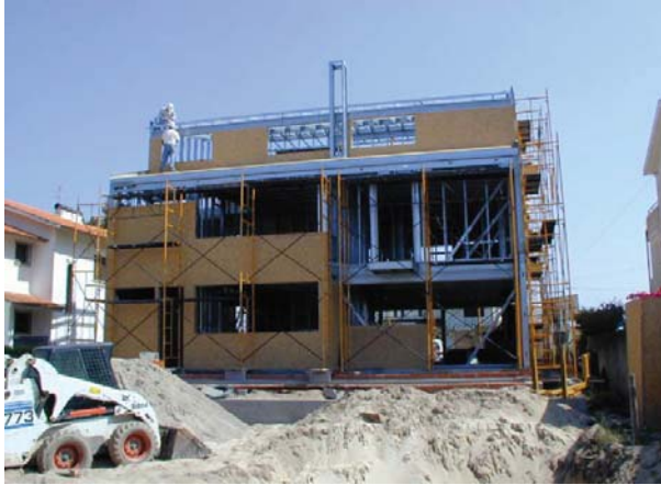
Figure 1. Light-weight steel frame
