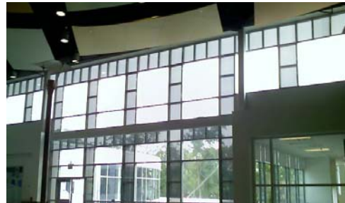
Figure 11. Photo of photovoltaic glass designed into atrium curtain wall
