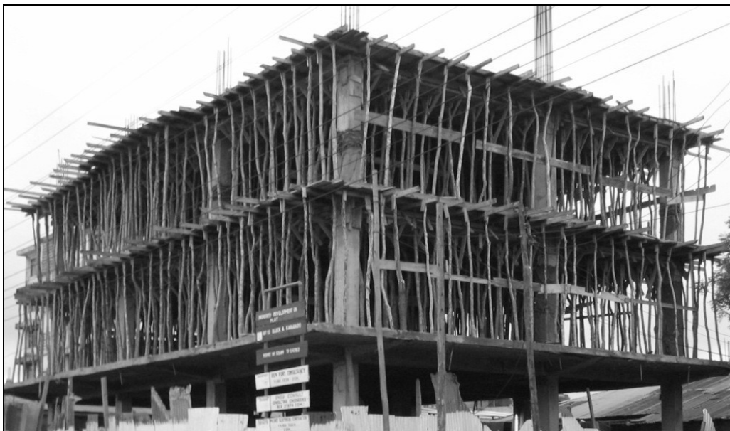
Figure 2. Typical wooden formwork used as temporary supporting structures in casting in-situ reinforced concrete in the construction of multi-storey buildings in Dar es Salaam City, Tanzania (field observation)
