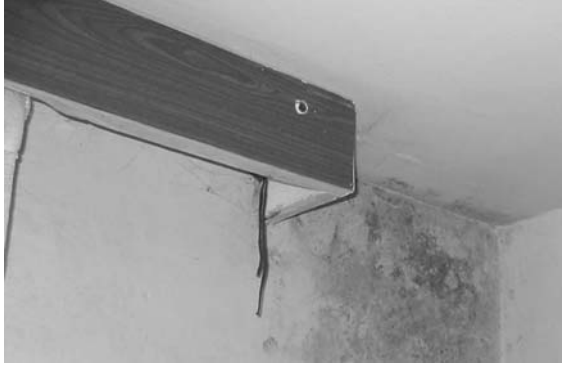
a. Mouldiness on the exterior walls
