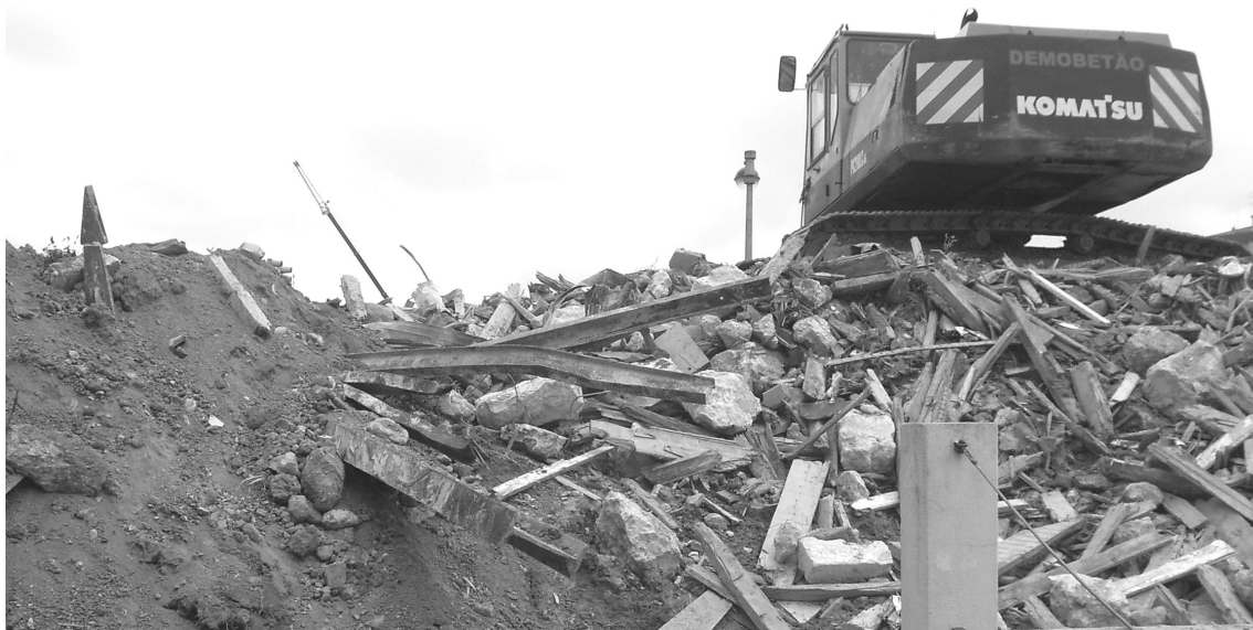
Figure 2. Typical early XX century building under demolition in Lisbon. Notice large percentage of soil content, with mixed metal, stone and wood elements
