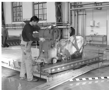
Figure 3. Processing of the de-mounted components with a concrete saw.
