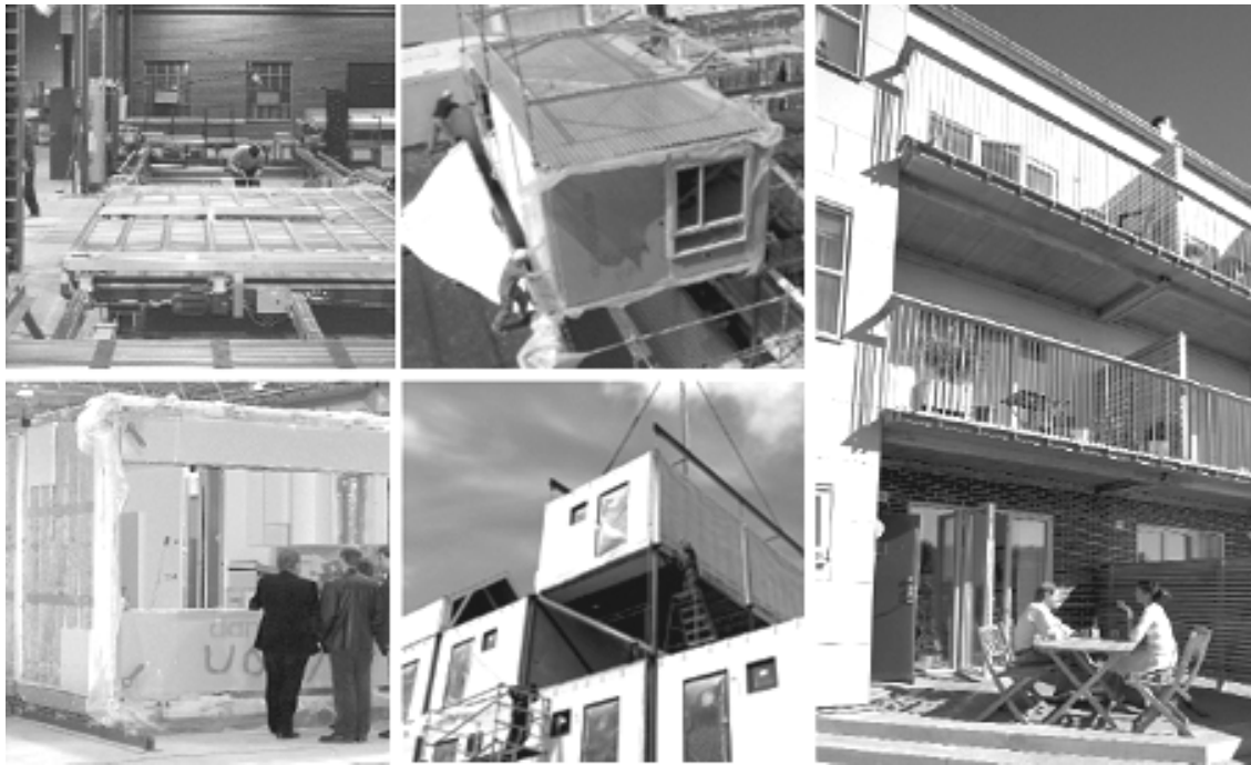
Figure 4. Application in Malmo (Sweden) of almost fully equipped modules in light gauge steel framing mounted in a framing system with steel columns to form multi storey residential buildings. The system provides cost-effective, environmentally sustainable dwellings of good quality and with short production time (Open House System).
