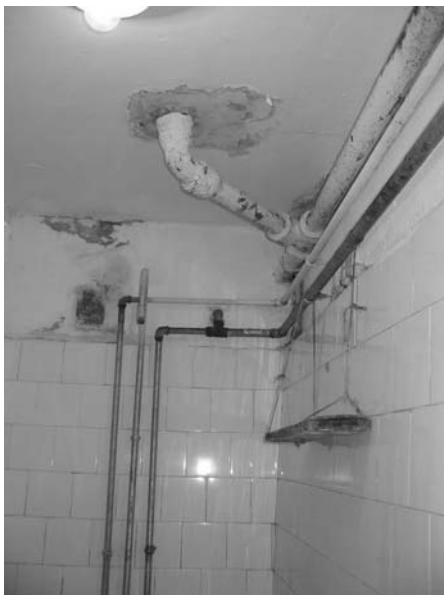
c. Degradation of the tiles and piping
