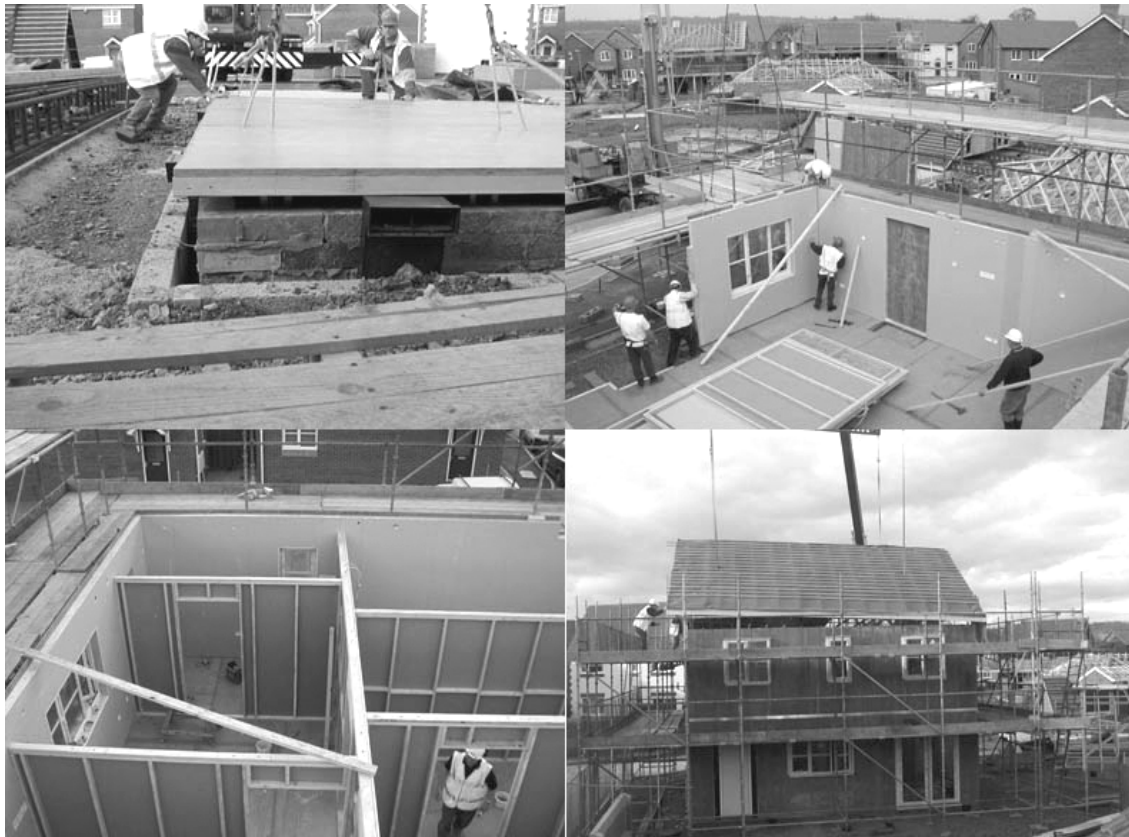
Figure 2. Structural timber housing system. Precision-engineered wall and floor panels are fixed together before the roof is lifted on to the top (Space4).
