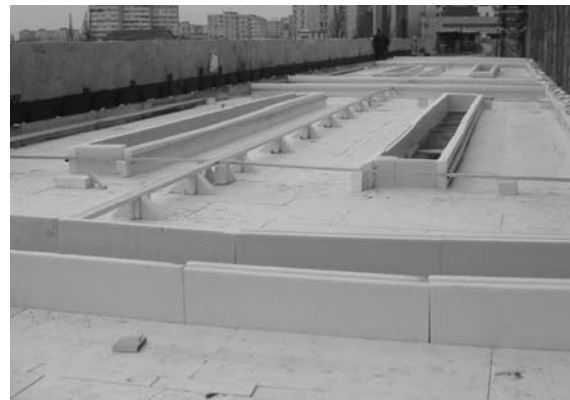
b. Terrace thermal protection
