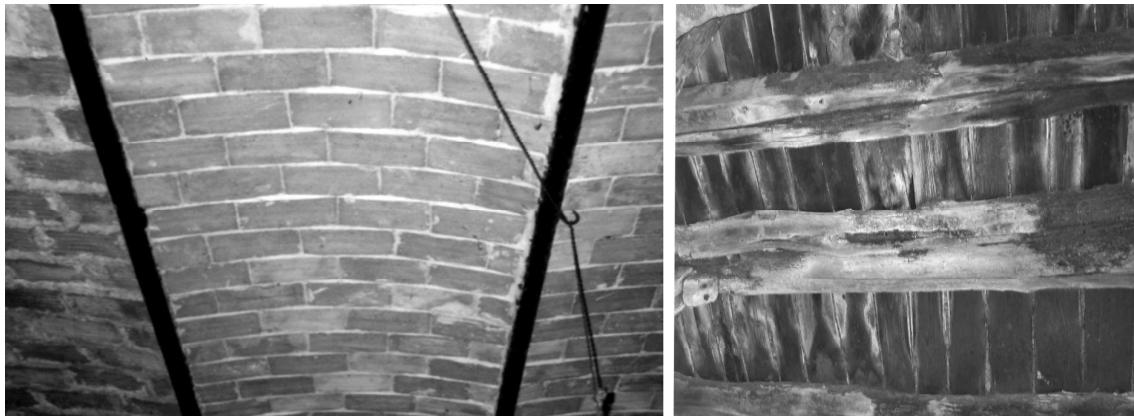
Fig. 3. The intrados of a floor supported by steel girders and a wood-floor.
