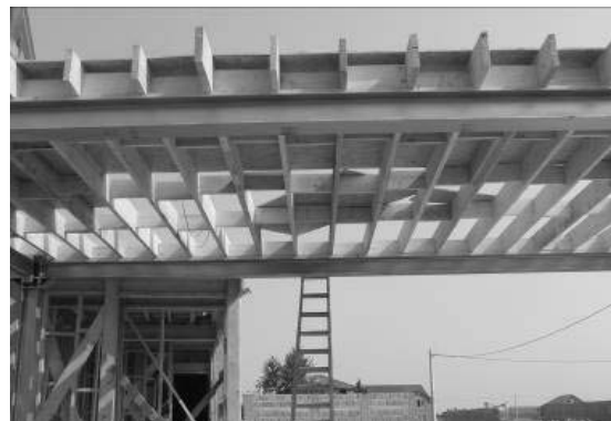
(b) the steel skeleton with timber floor
