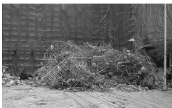
Figure 1. Sorted broken concrete and steel stockpiled separately (Guidelines for selective demolition).
