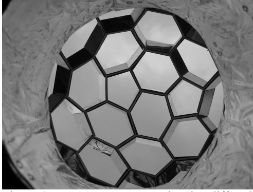
Figure 6 Transport component showing diffused light being reflected from capture component
