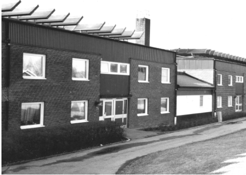
Figure 1. Ca 380 m 2 of solar panels added on two buildings in a housing area, in the south of Sweden. The panels are erected transverse the almost flat roofs, facing south and the sun as efficiently as possible. The solar energy is stored in two water tanks of 15 cubic metres each, and the heat is used for heating as well as hot water for the totally 120 flats in six buildings. The out effect is calculated to be 150 000 kWh.
