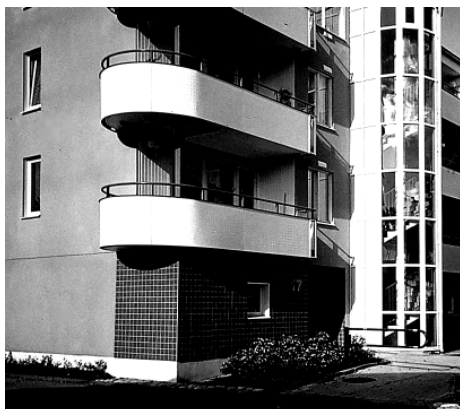
Figure 8. This building got a lift inside the original staircase and new stairs in an addition to the original staircase. Well insulating glass panels make the new staircase light and attractive. Enlarged balconies facilitate the use for disabled persons. The additions make the façades more vivid and expressive.
