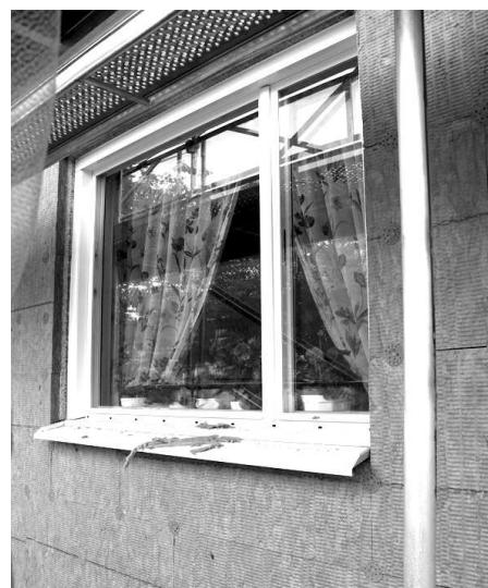
Figure 4 (left). The inner pane replaced by a sealed double-glaze panel. (Bjerking, 1987).
