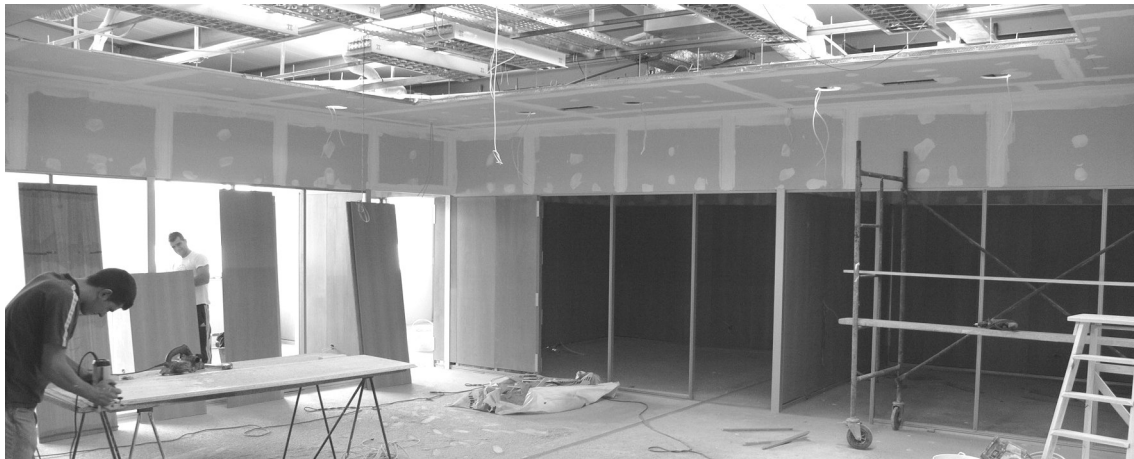
Figure 4. Work in progress at the new IP offices in Cacém (March 2006). Doors, wood veneer wall panels and all lighting fixtures were being reused after disassembly from original location in Lisbon.
