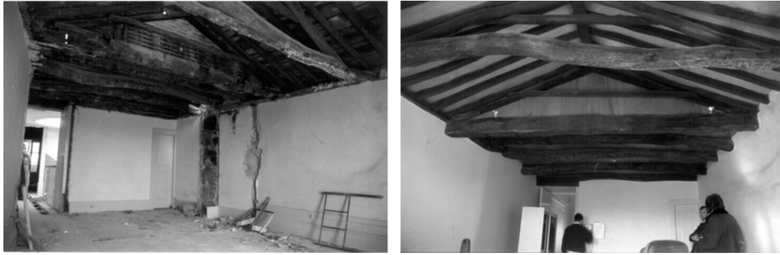
Figure 6. Interior of the wooden roof: (a) during deconstruction process and (b) after renewal.
