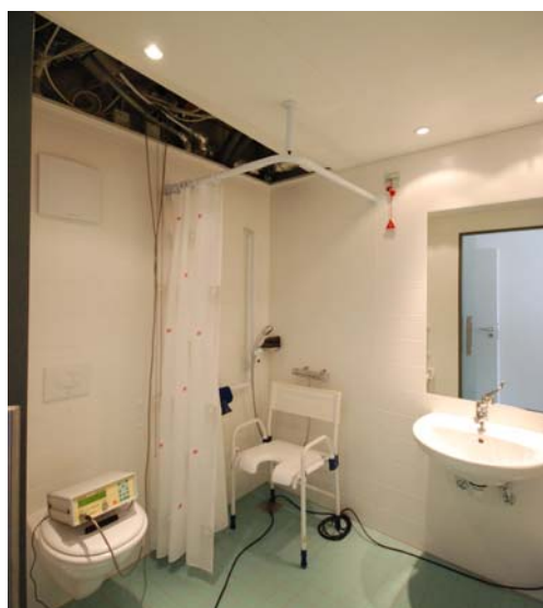
Figure 8 – Ultrasonic flow measurement
