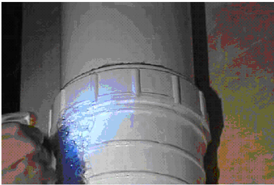
Figure 8 The leakage at the expansion joint was due to poor workmanship in applying PVC solvent cement.
