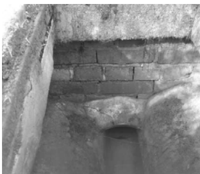
a. Damaged manhole joints
