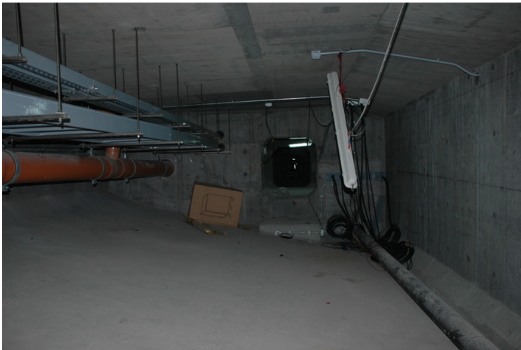
Photo 5 - Services housed inside “Tsing Ma Bridge”
