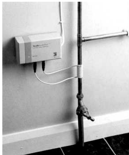
Figure 4 - Electromagnetic water treatment device
