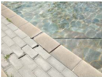
Photo-8 Crack of the ground in facility B
