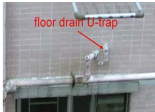
Figure 2 - Floor trap installed outside a building
