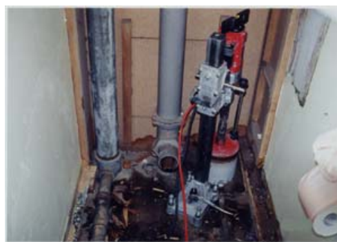
Photo 1 Updating work on the drainage stack and horizontal fixture drain branch in the privately owned section
