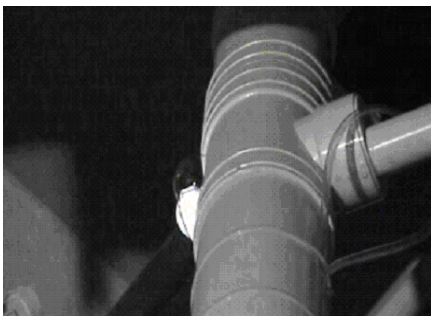
Figure 8 The leakage at the expansion joint was due to poor workmanship in applying PVC solvent cement.
