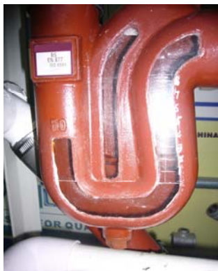
Figure 14 – Anti suction trap under positive pressure
