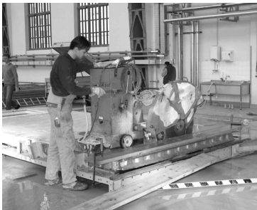
Figure 3. Processing of the dismantled components with a concrete saw.
