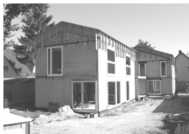
Figure 10. Building carcass of main and subsidiary houses completed.
