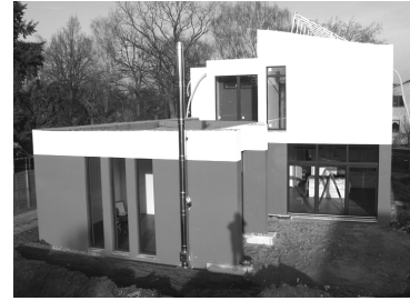
Figure 14. Building after completion.
