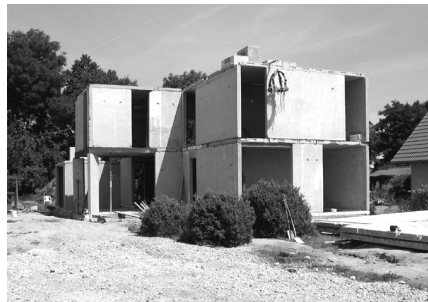
Figure 7. Building carcass after completion.
