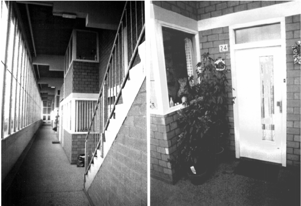
Figure 6: Internal view (DWL, Pi de Bruyn)
