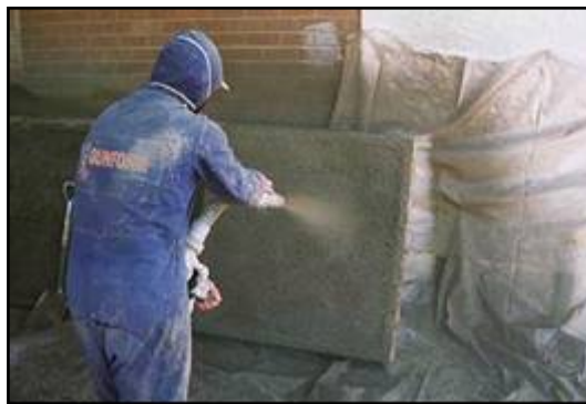
Figure 2. Spraying distance and angle were kept around one meter and 90°, respectively.
