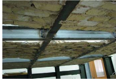
Figure 2. Two way method retrofitting jack arch slabs
