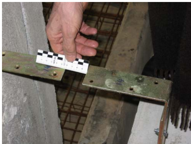
Figure 8. One sided shortening of the floor slab by 38mm
