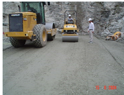
Figure 12. View of spreading and compaction of RCC in Jegin dam
