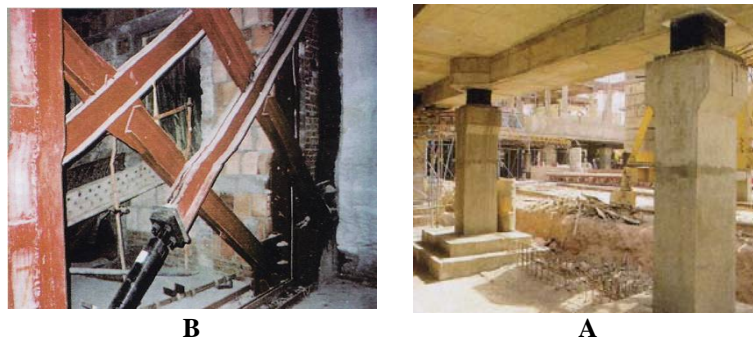
Figure 1. Kinds of mechanical damp ions a) pillar. b) Bracing Rod
