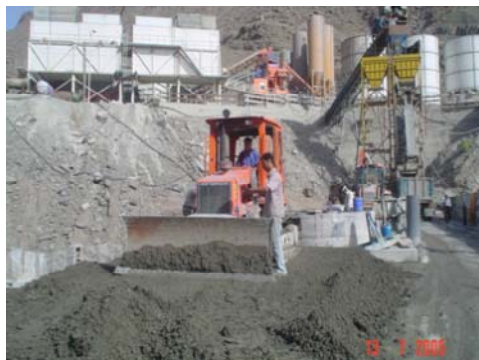
Figure 12. View of spreading and compaction of RCC in Jegin dam
