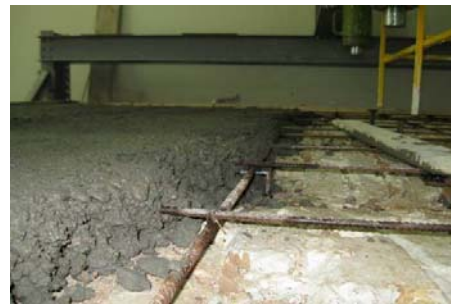
Figure 1. Concrete layer method for retrofitting jack arch slabs
