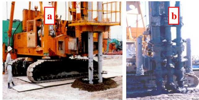
Figure 3: (a) The CDM machine with 2 augers (b) The CDM machine with 3 augers
