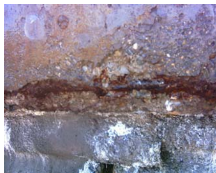
Figure 4. Severe corrosion of reinforcement
