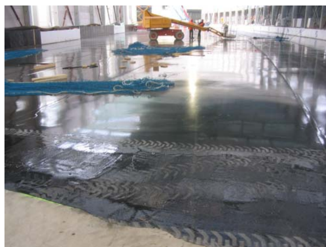
Figure 5. The smoothness of the bitumen layer on top of the sub-concrete
