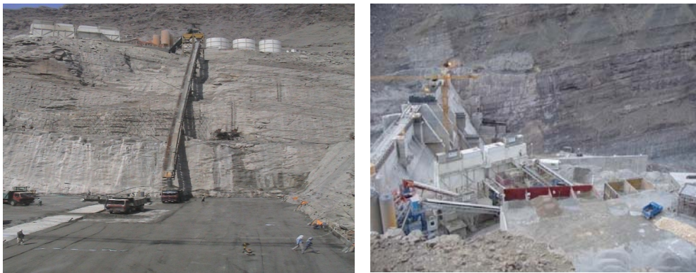
Figure 11. View of vacuum chute used at Jegin dam and general view of site lay out
