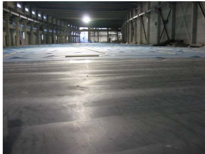
Figure 10. The glass like surface of the finished concrete slab
