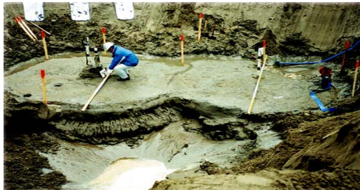
Figure 10. The soil cement columns which have been made by ras-jet system
