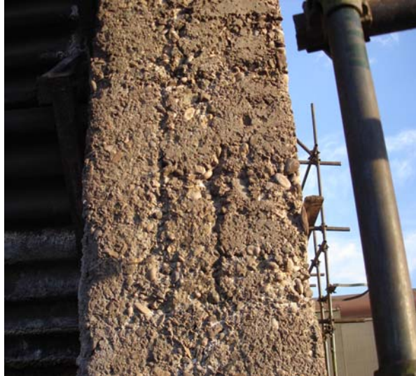
Figure 5. Removing of cement paste and exposed aggregates
