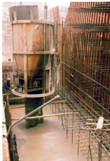
Figure 4. Orifice concreting
