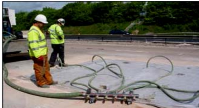
Figure 8. The plastic cover is used for all air to be sucked into any void spaces as well [12]
