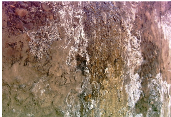
Figure 6. Leakage and efflorescence
