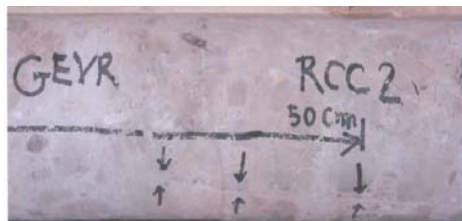
Figure 8. Typical transitions between GEVR and the RCC (24 hrs. joint)
