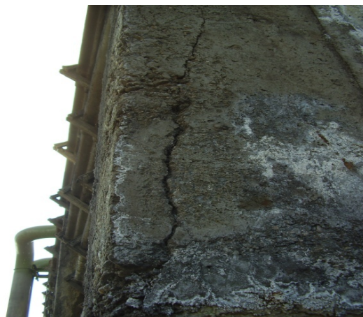
Figure 3. Longitudinal cracking and sulfate attack
