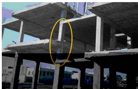
Figure 1. Short columns mentioned duplex reinforced concrete [16]
