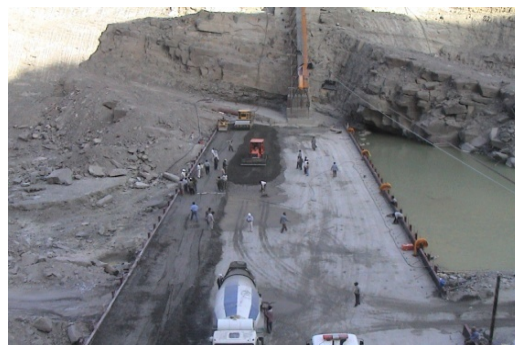
Figure 7. Photograph of RCC placement in coffer dam at Jegin with chute in background
