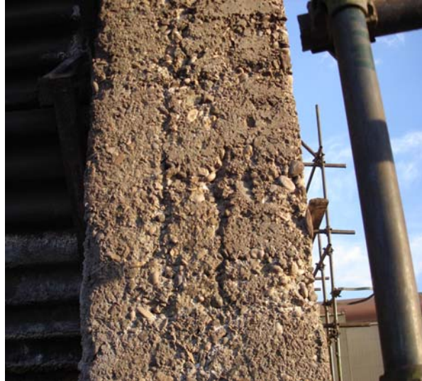
Figure 5. Removing of cement paste and exposed aggregates
