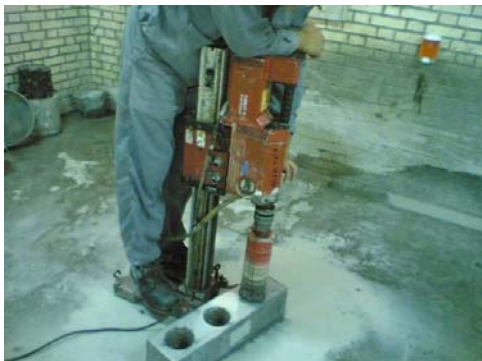
Figure 2. Coring of beams
