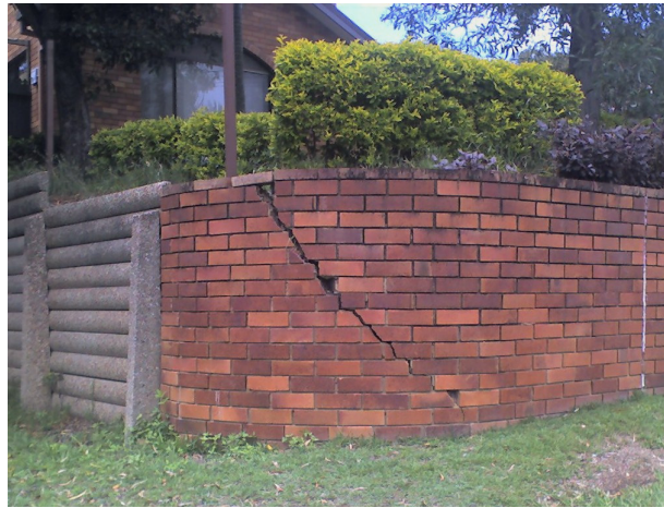
Figure 1 Failure of a domestic retaining wall due to earth pressure.
