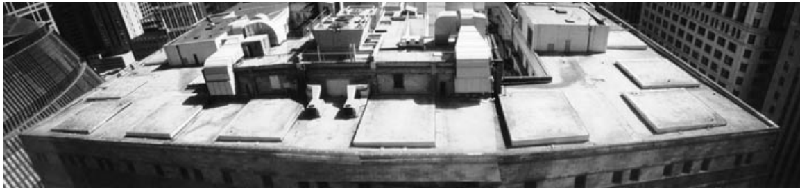
Figure 1 Aerial view of the Chicago City Hall roof top's existing condition in 1999.
