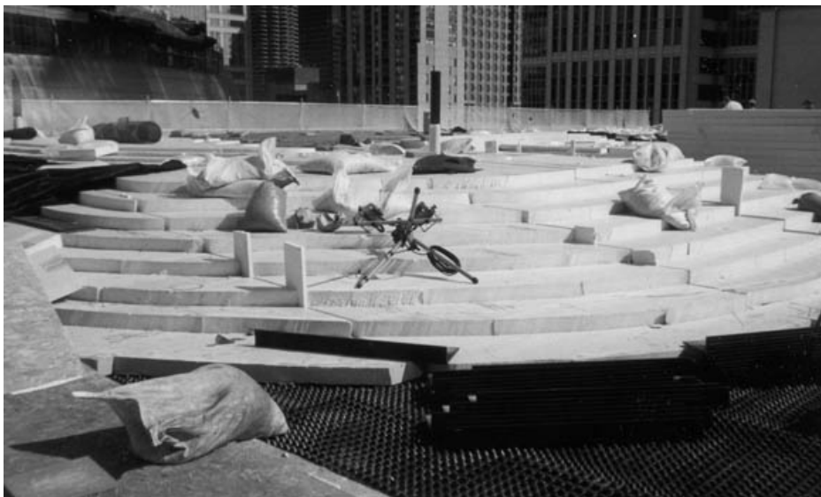
Figure 7 Rolling topography was created with stacked layers of extruded polystyrene.
