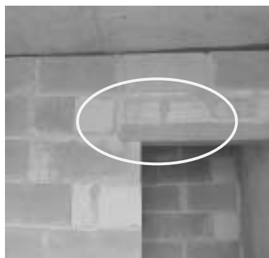
Figure 6 – Concrete blocks cut on top of door.
