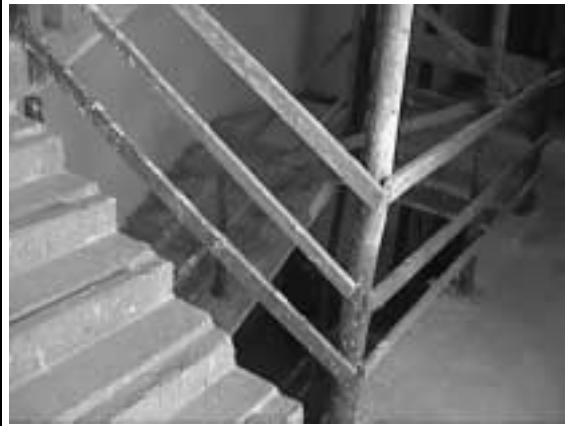
Figure 04: Temporary closing of the opening and steps of the stairway, of 1,20 m of height, constituted of fixed resistant material to the structure.
