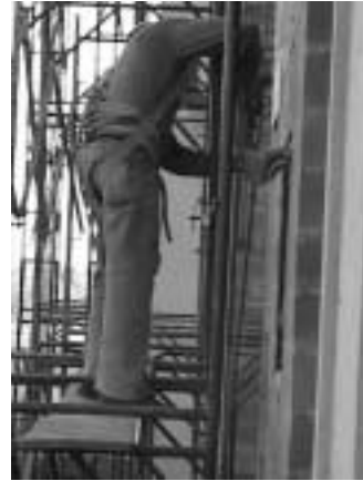
Figure 08: Details of worker accomplishing service in scaffold to facade and using safety belt. However, the placement of the boards for formation of work floor is precarious and insecure.
