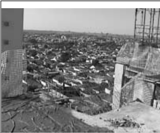
Figure 03: Protection for screen installed in the last flagstone where the risk of workers' fall and projection of materials exists.
