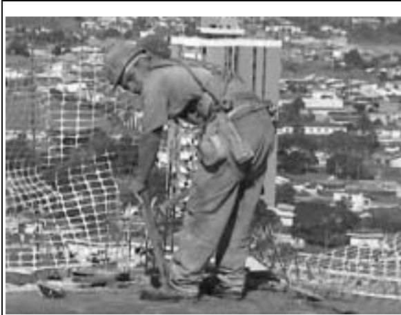
Figure 07: Worker accomplishing service in the last flagstone of the building, prisoner to the safety belt type parachutist, obligatory for accomplished activities the more than 2 meters of the floor.
