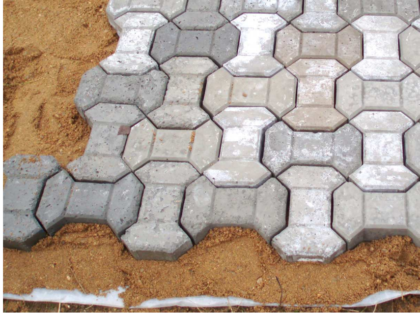
Fig. 2. Application of block pavement from alkaline-activated fly ash on sand bedding
