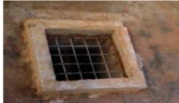
Fig. 9. Shows the roof opening
