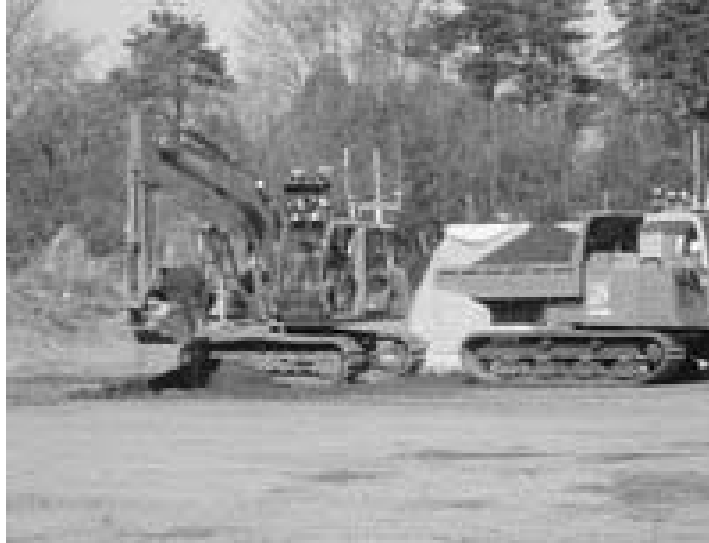
Figure 6. Excavation and Loading
