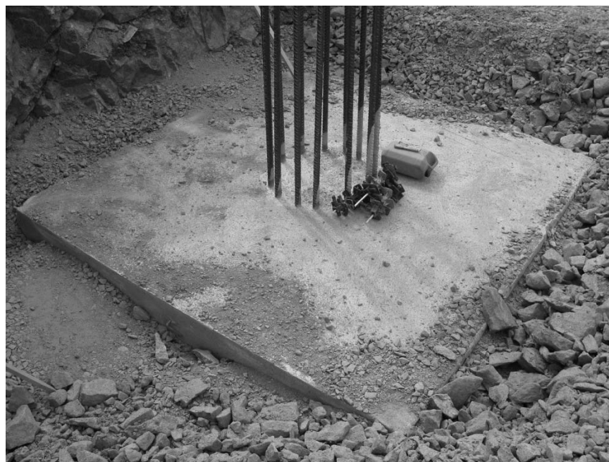
Figure 6. Finished bridge foundations, partially covered in gravel.
