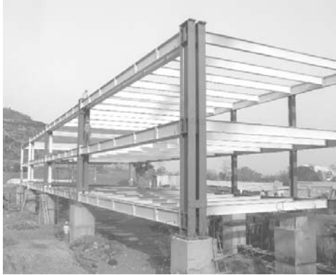
Figure 4: Erected Frame after 1st Lift
