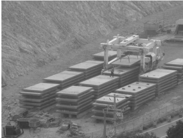
Fig. 3. Precast concrete panels
