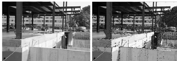
Figure 3. (a) An image taken on 09/27/08 from Student Dining and Residence Hall projects; (b) Same image in grayscale with SIFT feature locations visualized in blue
