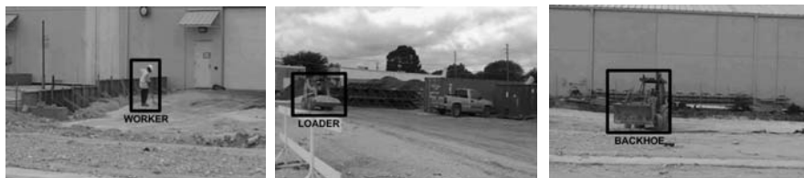
Figure 6 Object identification and tracking: worker, loader, and backhoe
