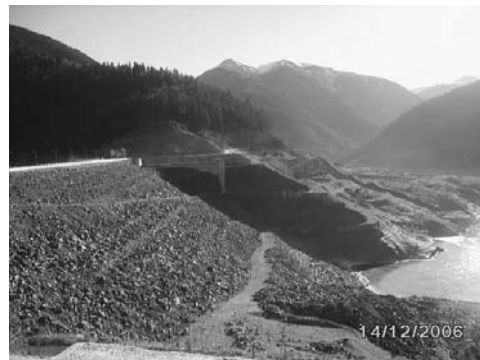
Figure 1. View on the Gura Apelor Retezat Dam
