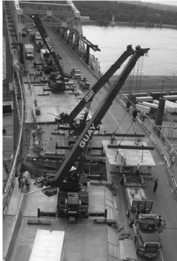
Figure 1: Groups of cranes working on a bridge
