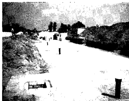
Fig. 2. Foundations, basement floor and piping being laid before construction of the cellar.
