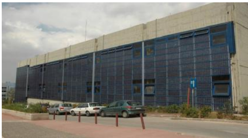
Figure 1 Building façade with the first six PV arrays
