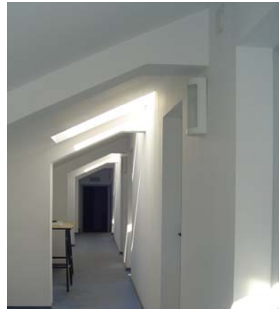
Figure 4 The attic of the School of Architecture, before the work of refurbishment and after; the volumetric and imagistic features of the building are preserved, by using the same type of roofing material (ceramic tiles), but the use of the interior space has changed, from technical to functional
