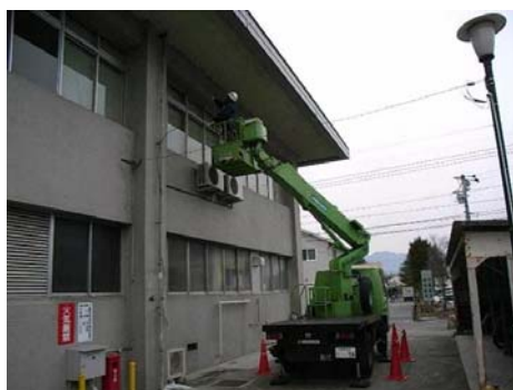
Photo 1 hammer test
