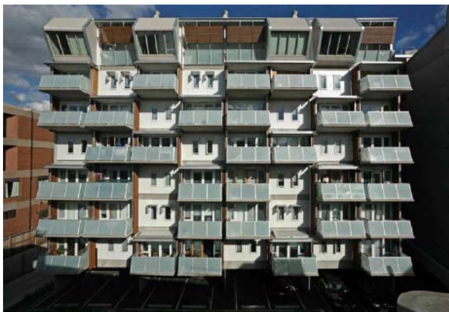
Figure 2 North elevation of rear building block showing solar shading and balconies (© Peter Hyatt)
