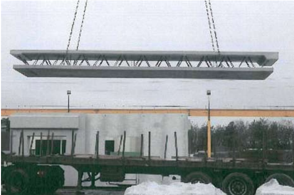
Figure 13 New type of concrete double floor has an extraordinary span of 18 to 20 meters
