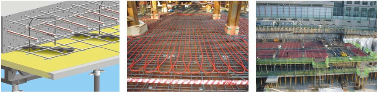
Figure 8 Detailed schematic diagram of CCA and construction pictures of CCA pipes
