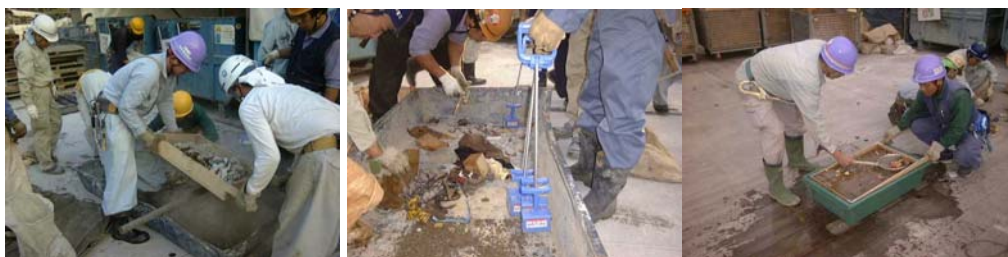
Figure 7 Images from Zero Emission activities, sand strainer, screen out woodchips, metals, etc. (left), magnet, pick up metals either by large magnet (center) and water, classify woodchips out from floats (right).
