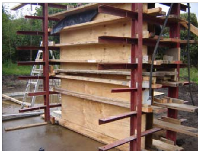
Figure 4 Photograph of the modular Uku formwork system developed by the research team
