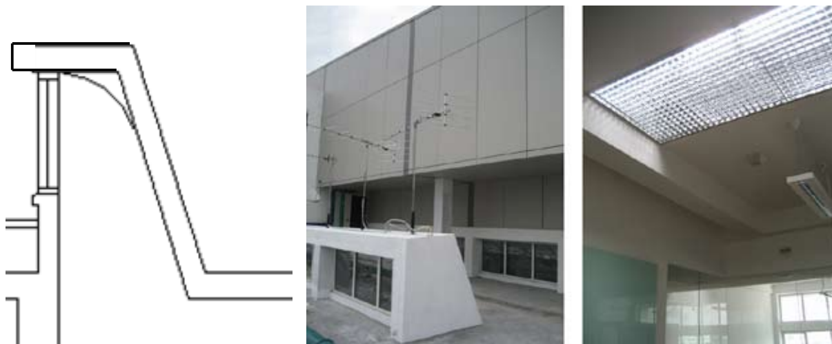
Figure 10 Roof lights oriented to the north photographed outdoors and indoors
