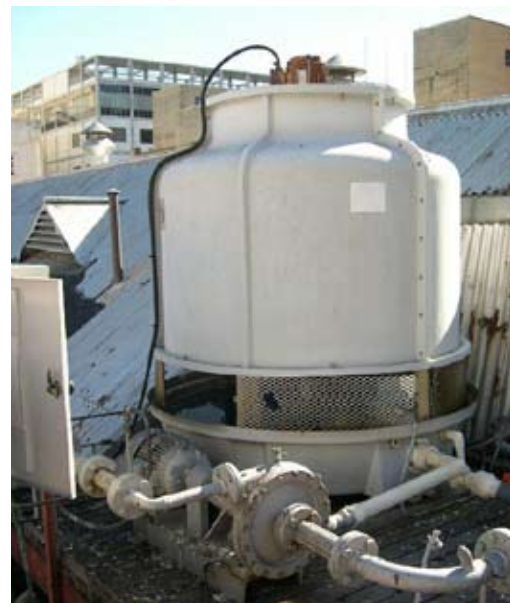
Fig 7 old cooling towers pose potential health problems and are high in maintenance costs
