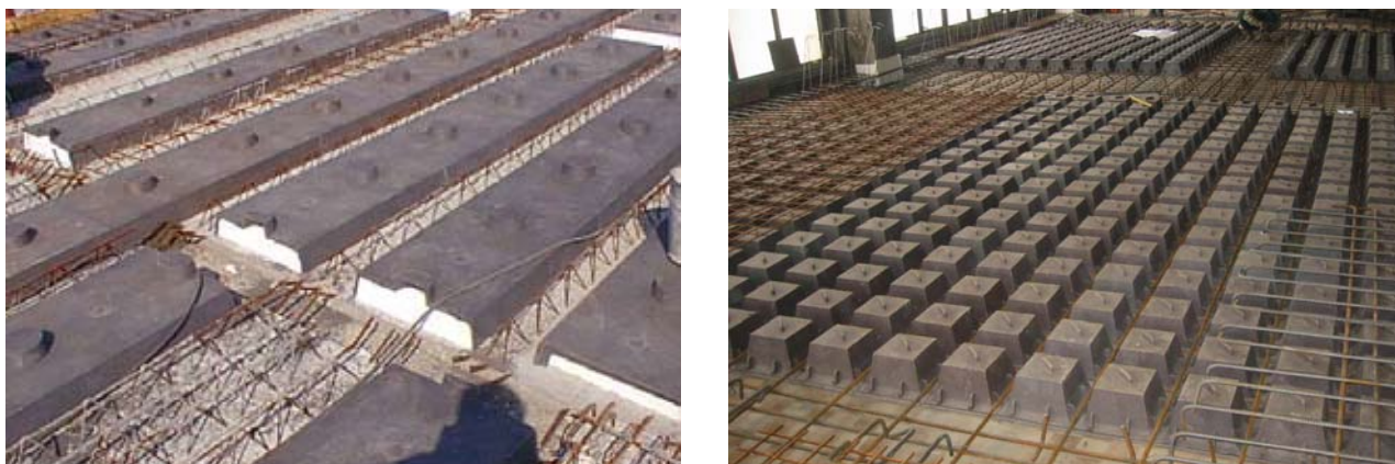
Figure 7 a - Construction of Senior Centre Moravany – composite RC slab lightened by installation fillers from recycled non-sorted plastic from municipal waste, 2000, b - Reconstruction of floor slab in Skoda factory hall. Slab is lightened by waffle fillers from recycled non-sorted plastic, 2003-2004
