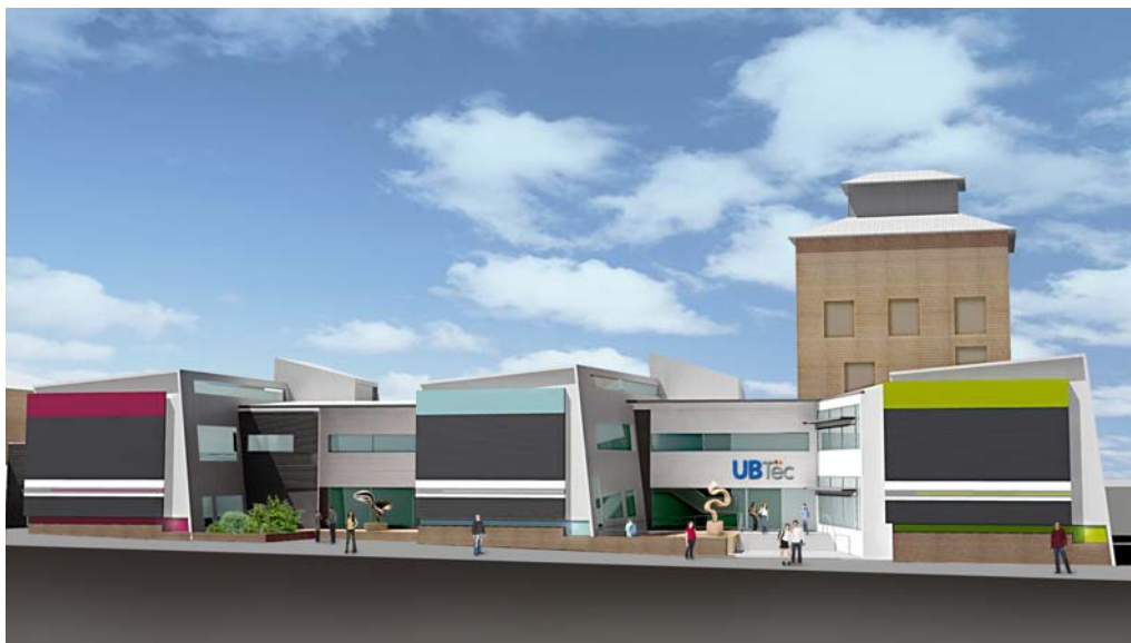
UBTEC. Image courtesy of the Architects Gray Puksand. Note the large solar air heaters on the end façades.
