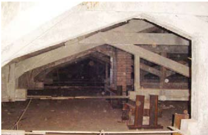
Figure 4 The attic of the School of Architecture, before the work of refurbishment and after; the volumetric and imagistic features of the building are preserved, by using the same type of roofing material (ceramic tiles), but the use of the interior space has changed, from technical to functional
