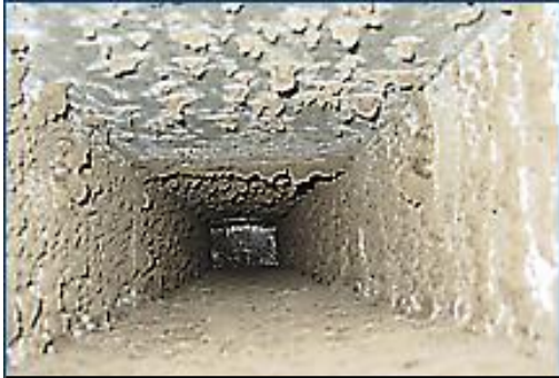
Fig 6 Dust and mould growth accumulate inside ducts
