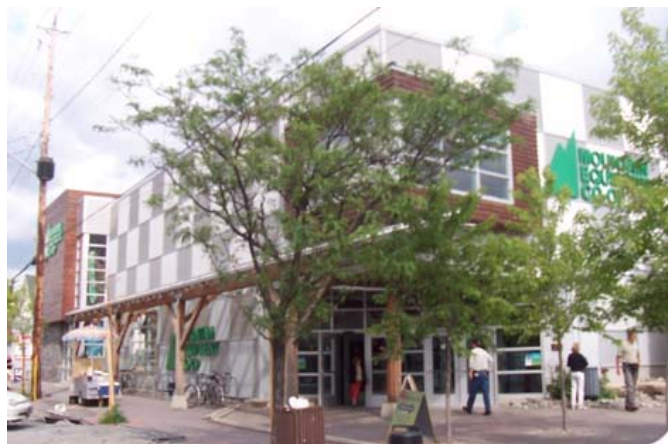
Figure 1 In Canada the Mountain Equipment Coop has pioneered component reuse in many of its retail stores. This one located in Ottawa reused many parts of the previous building on site, including the foundations..
