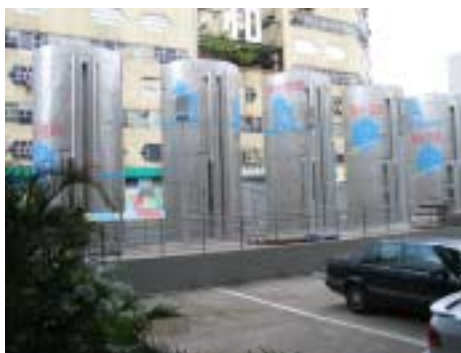
Figure 7 Ice storage tank at the entrance of the building
