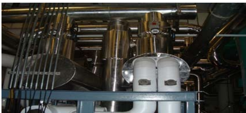
Figure 5 The renovated ice chiller with its evaporator replaced and turned into a brine chiller in the NMMB project
