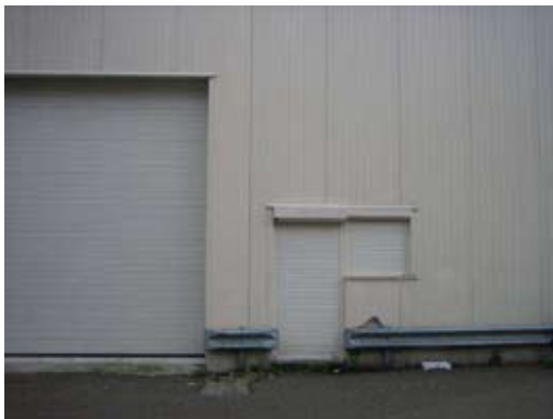
Figure 1 Sandwich panels, Doors and windows in the existing situation.
