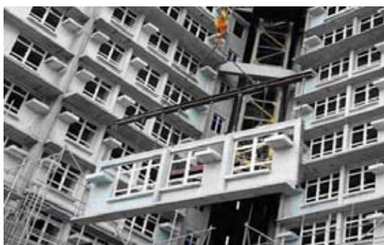
Photo 5: Increased Use of Pre-cast Concrete and Prefabricated Elements in Building Construction Works
