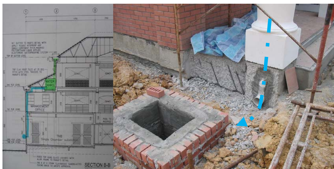
Figure 10 from left – construction detail showing water harvest system at the community center & Rain water downpipe and the collection sump under construction
