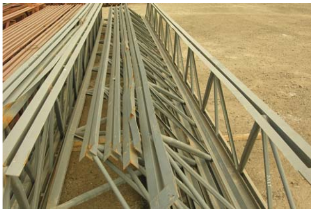
Figure 3 Open web steel joists can often be dismantled for reuse, but the new structure needs to be designed around the available spans.
