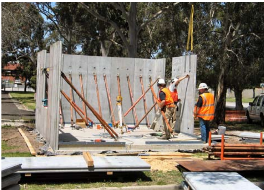
Figure 5 Precast LBCM panels being lifted and propped.
