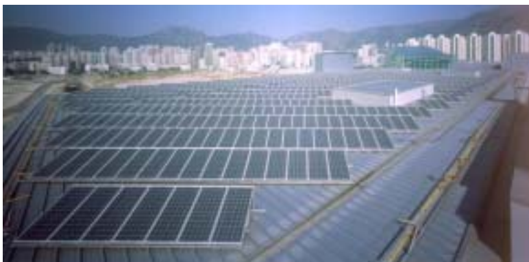
Figure 2 Photovoltaic Panels installed at the roof of the building
