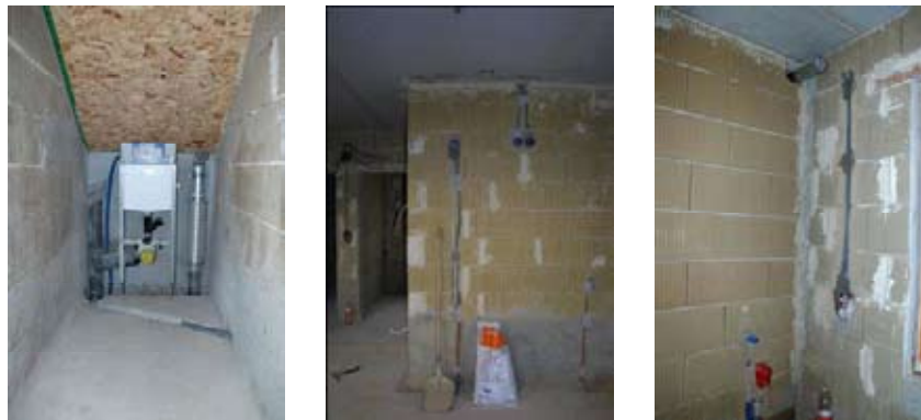
Figure 7: Water pipes are mainly led into the floor. Installation lines in the unfired loam brick walls are not a problem.
