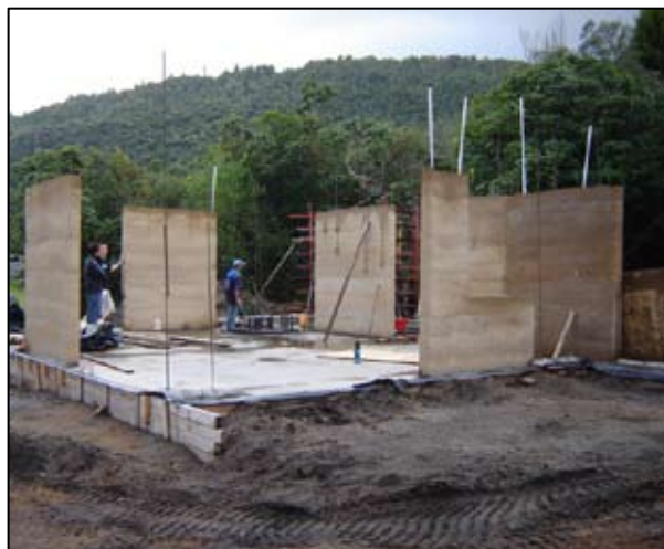
Figure 6 Uku dwelling in Rotoiti under construction.
