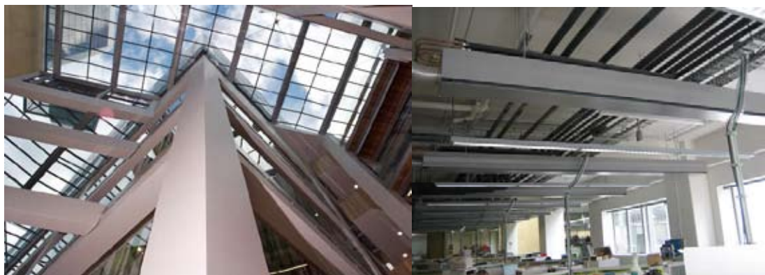
Figures 1 and 2: Pictures of the Department of Conservation's new head office with the atrium on the left and chilled beams on the right (Source: Pictures courtesy of the Department of Conservation)
