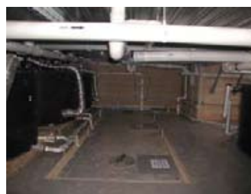
Figure 3 From left: composters, leachate storage tank and urine tank.
