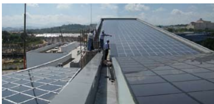
Figure 1 Zero Energy Building photographed from entrance and at photovoltaic roof
