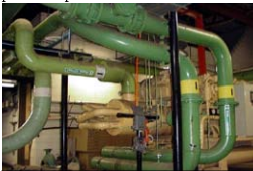
Fig 5 Typical old chillers are inefficient and often contain ozone depleting substances
