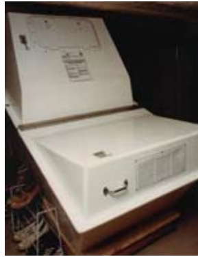
Figure 1: composting WC operated by hand.
