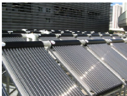
Figure 4 Evacuated tube types solar collectors installed on the roof of vehicle reception office building
