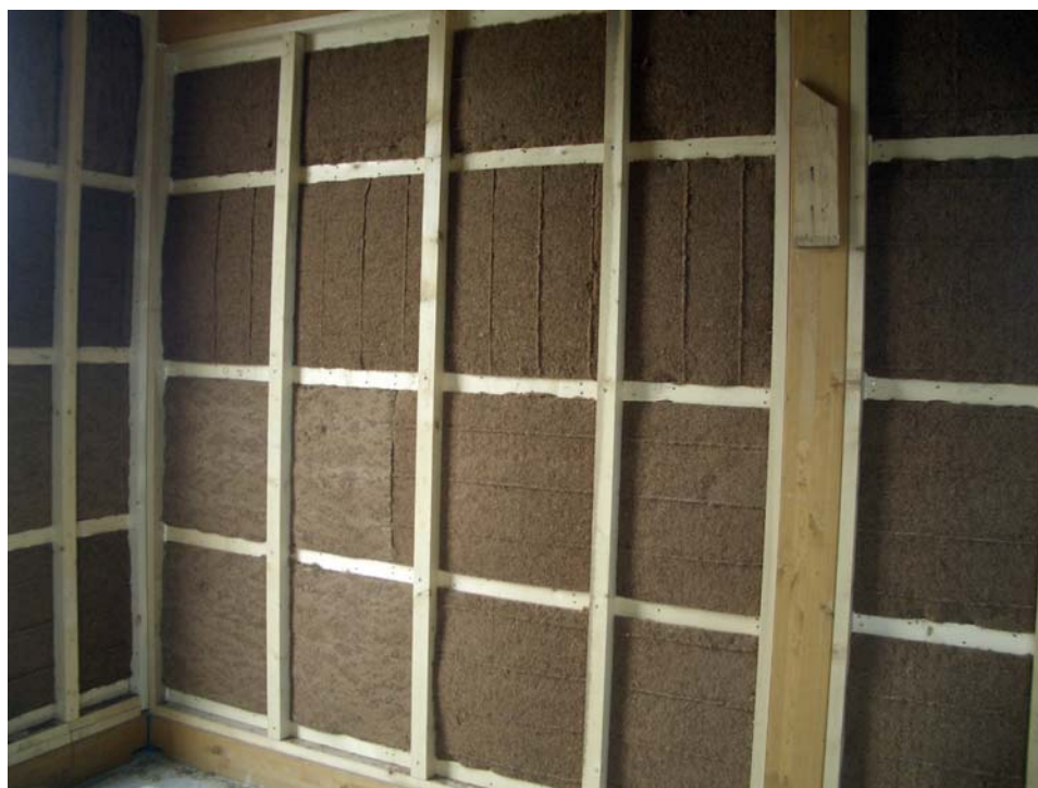
Figure 4 Picture of the inner part (main wooden frame) of the external wall under construction
