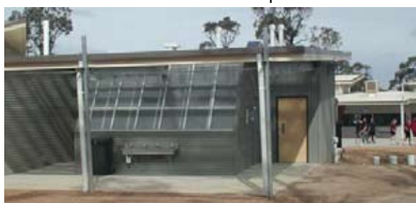
Figure 2 The urine-separating dry composting toilet block and greenhouse enclosure.
