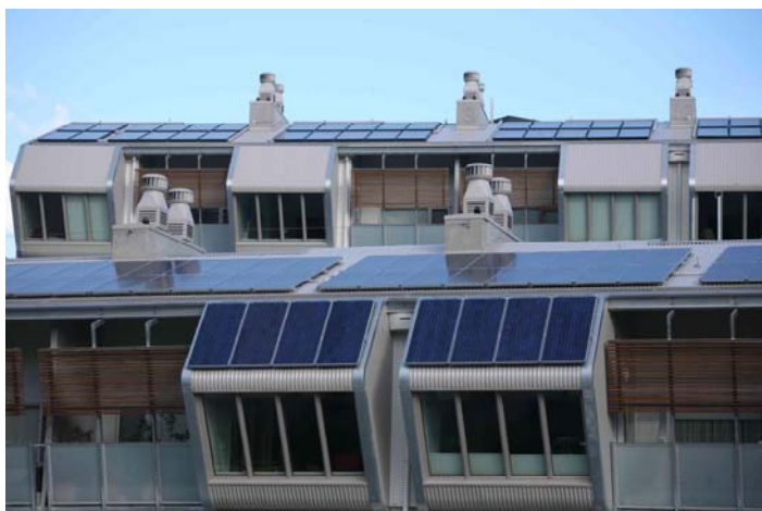
Figure 4 Image showing photovoltaic panels (foreground), solar thermal collectors (background) and wind ventilators on exhaust risers. (© Peter Hyatt)
