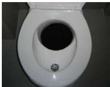
Figure 4 One of the urine-separating pedestals.
