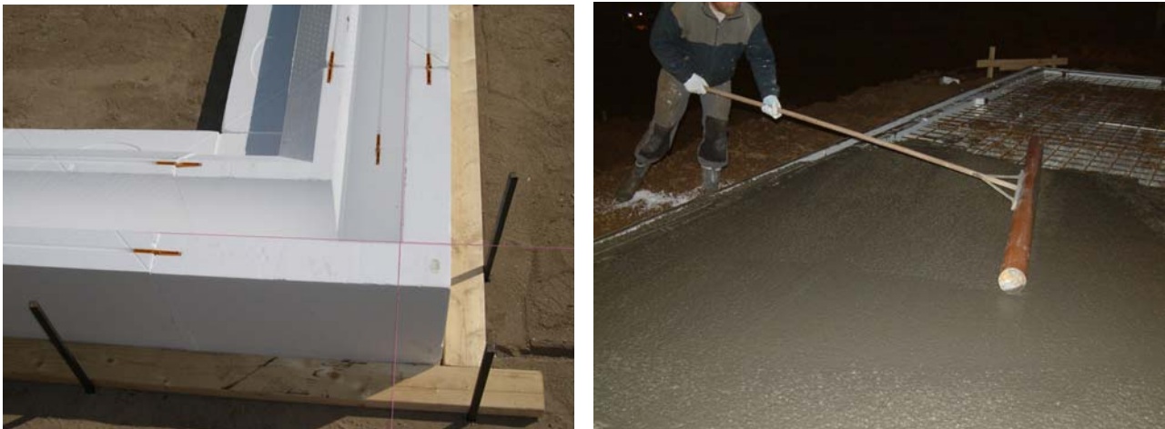
Figure 6 a): Left, prefabricated lightweight elements, made of EPS, mounted as the strip foundation. The elements were fixed together with large clamps of plastic, b): Right, 300 mm EPS, mounted as two layers on top of the base of stamped gravel bordered by the strip foundation that served as the insulation layer underneath the concrete floor slab. Iron was mounted as a net inside the strip foundation and as wires along the moat formed by the two vertical boards of EPS in the prefabricated elements, before concrete was cast and leveled.
