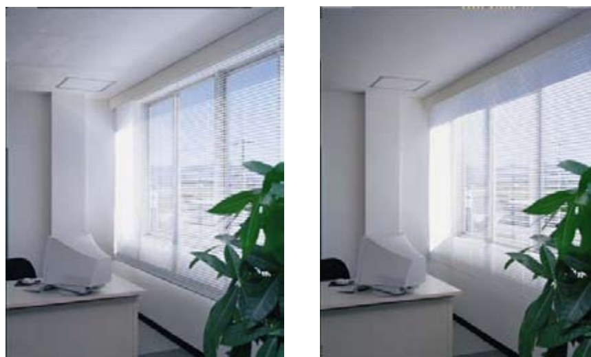
Figure 8. Ability to view outside The difference between “Gradation Blind” (left) and conventional blind (right)
