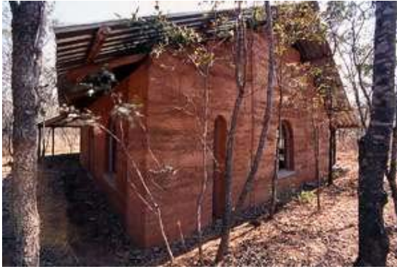
Fig 14. Rammed earth DfID block at SIRDC, Hatcliffe, Zimbabwe. Source: In Situ Rammed Earth Co. Ltd, Zimbabwe, 2005
