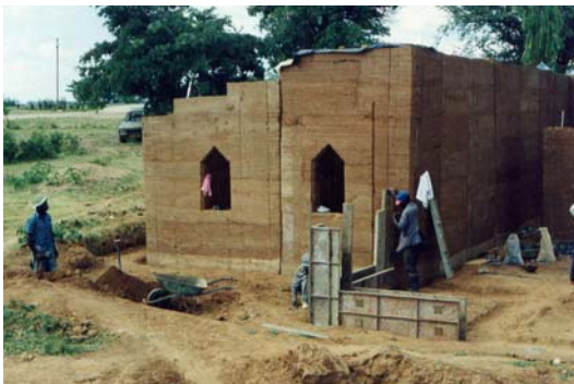
Fig 16. Chimanda House under construction Source: In Situ Rammed Earth Co Ltd (2006)
