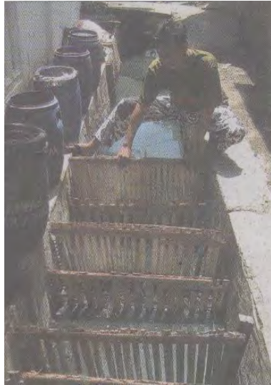
Figure 7: Traps are placed in the drainage to trap the mud in three phases (Source: Jawa Pos, July 14, 2008)
