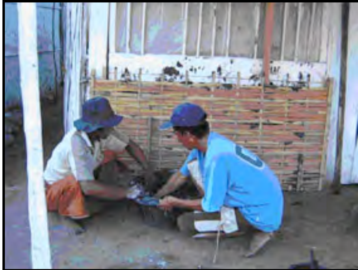
Figure 9 Casting of mud salt wall
