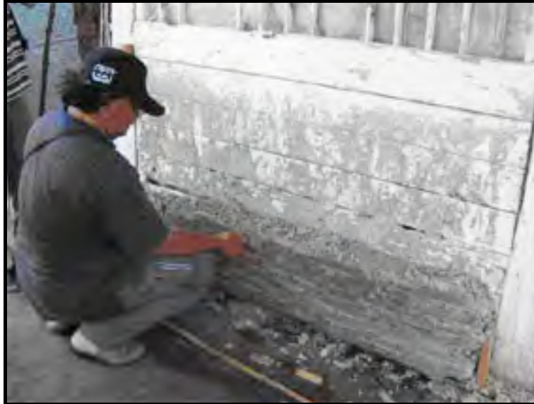
Figure 11 Salt mud wall after the casting is open
