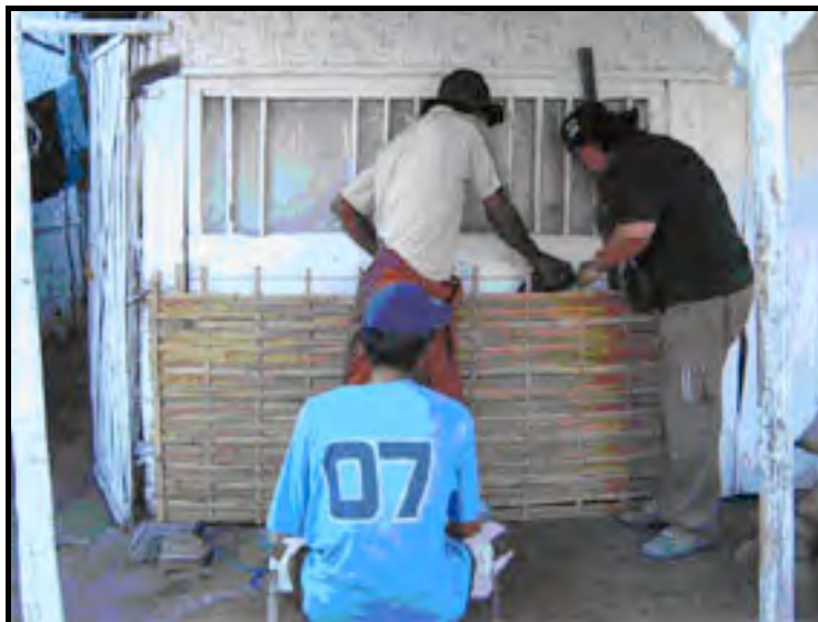
Figure 10 Compacting mud salt into cast wall
