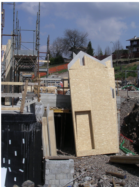
Fig. 8 Prefabricate wall panels before the construction phase
