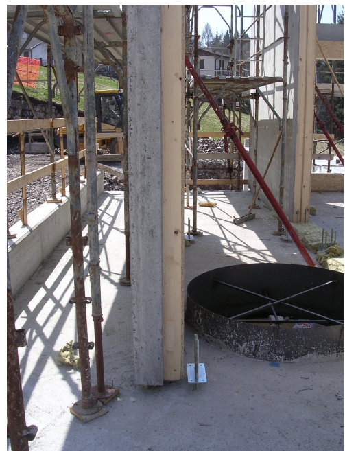
Fig. 9 Construction phase: prefabricate wall panels installed under de concrete floor
