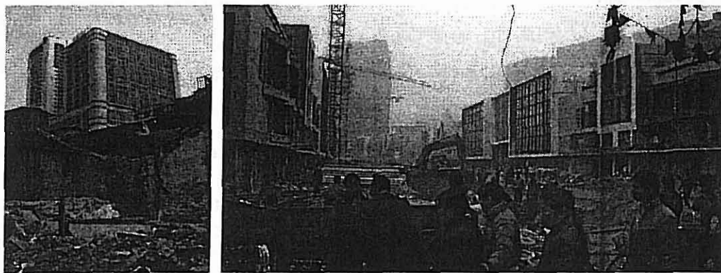
Figure 1: Urban renewal project “No.1 Ave. of Hanzhengjie Area”
