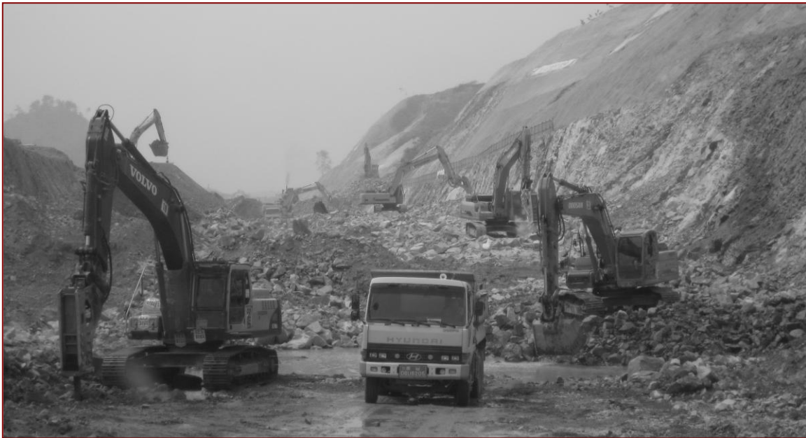
Figure 1: A typical job site configuration
