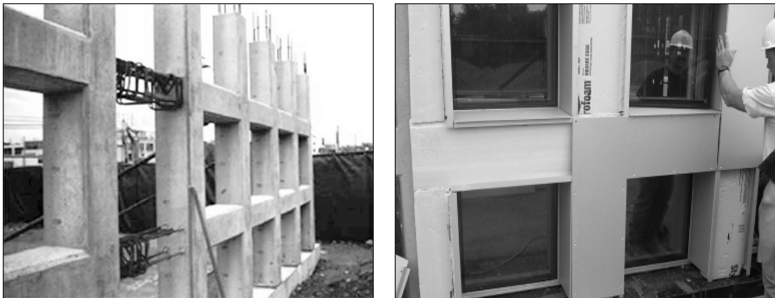
Figure 5 (left): The wet joint connection under construction
