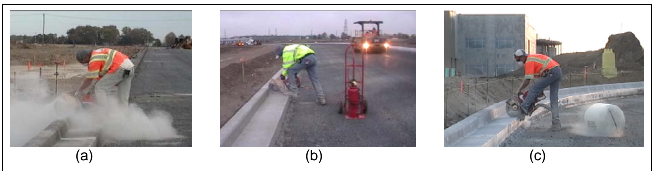
Figure 1: Concrete cut-off saw methods: a) Dry method b) Wet method c) LEV method.
