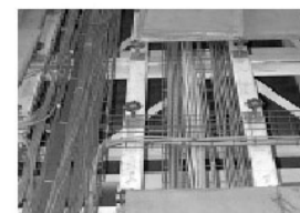
Detail of Grid (power, voice, data, video) distribution in the IW
