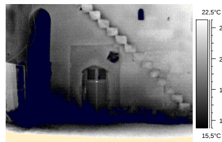
Fig. 6: Infrared image of the view shown in Fig. 5
