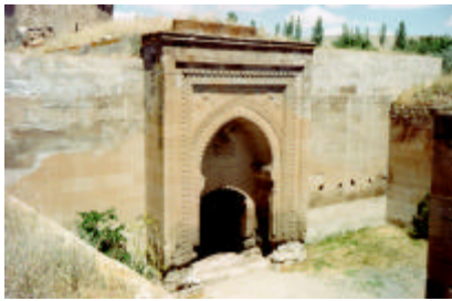
Fig. 1: General view of the north elevation at the courtyard, Agzikarahan
