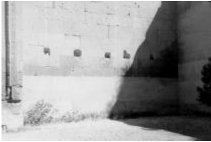
Fig. 12: Partial view of the lower parts from the north elevation at the courtyard
