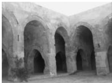
Fig. 7: Partial view of the south and west elevation at the courtyard
