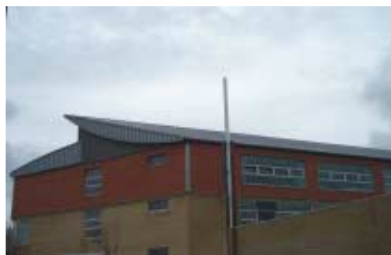
Figure 7 – Collecting roof for rain water
