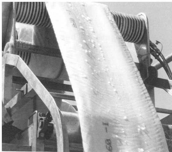
Figure 5 – Installation of the liner (soaked with reaction resin): for an exact placement through sewer manhole
