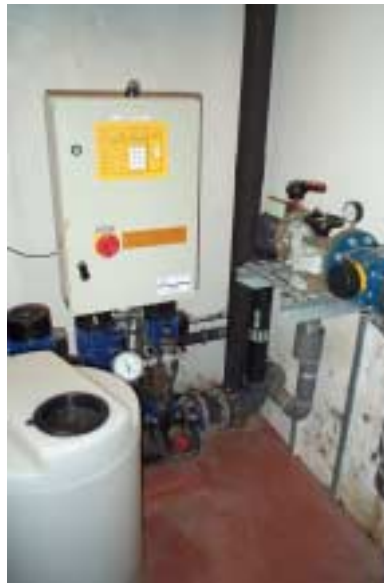
Figure 8 – Chloration system
