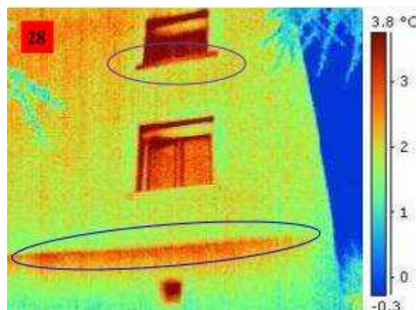
Figure 3. Infrared thermography performed after the renovation
