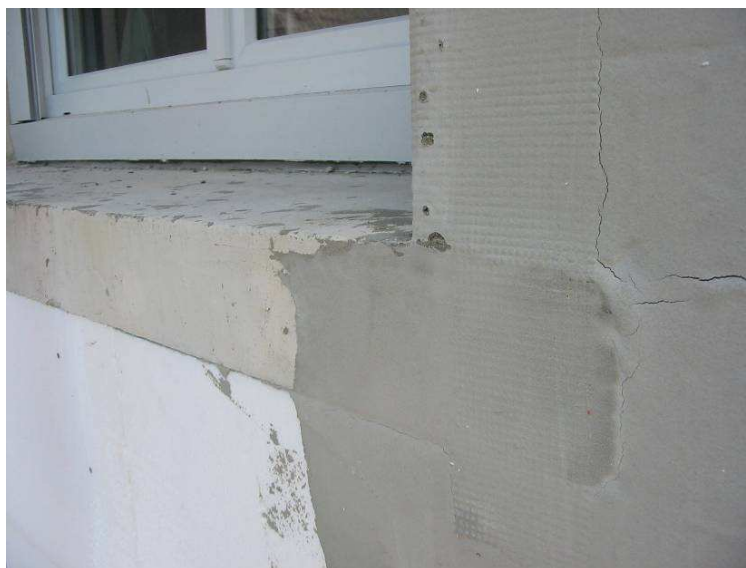
Figure 2. Treatment of windowsills in a renovation
