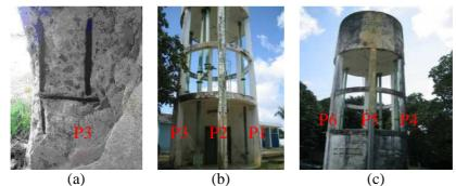
Figure 3. Visualization of pathologies from the 20 years old reservoir structure.
