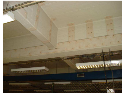
Figure 6. Reinforcement beams and pillars - 2008.
