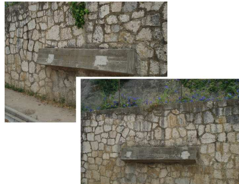
Figure 4. Micro-piles head block - 2008.
