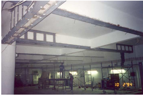
Figure 5. Metallic reinforcement beams and pillars - 1991.
