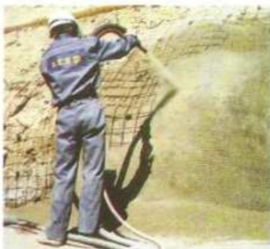
Figure 3. Sprayed concrete - 1991.
