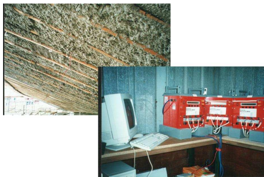
Figure 7. Norcure desalination system in operation - 1998.
