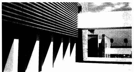
Figure 2: CHSC. Concrete louvers over east facade.
