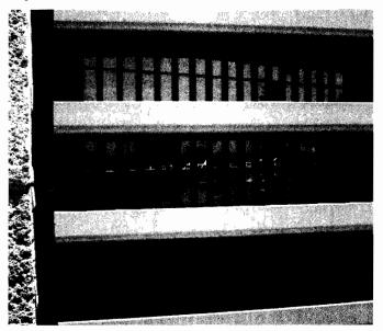
Figure 3: CHSC. Aluminium louvers over south facade.
