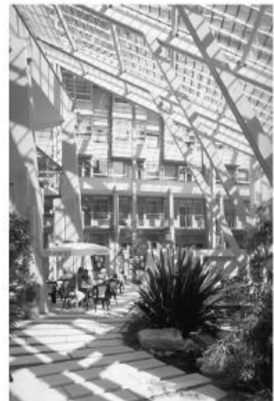
EARTH PORT Tokyo Gas, Japan Design philosophy of the Tokyo city gas supply company office building addresses "life cycle energy saving" by energy conservation and by optimizing natural ventilation and daylighting. Remarkable reductions of energy consumption and operating cost have been paid by moderately increasing initial cost.
