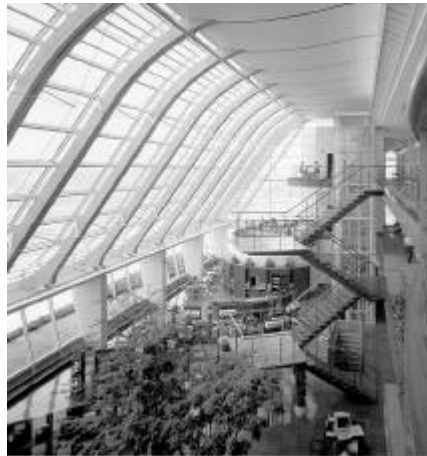
Atrium building concepts provide attractive spatial amenities for occupants and benefit from energy and environmental qualities: below: PRISMA ATRIUM, Germany
