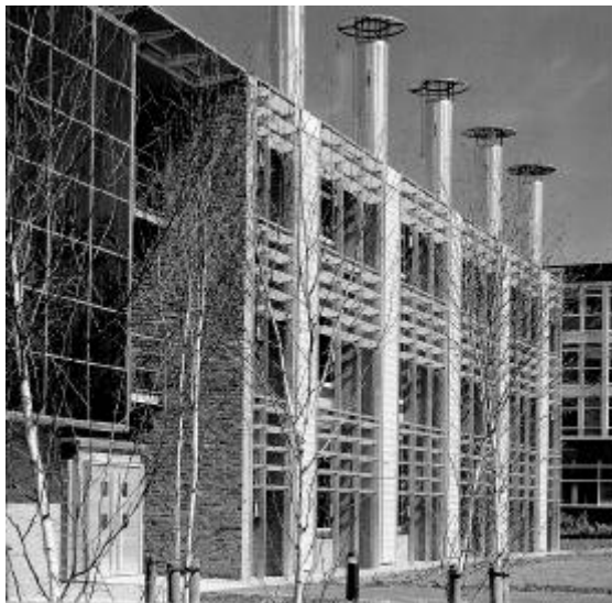
BRE Environment Office, Garston, U.K.: Highly engineered future role model for environmental office design. The building had been pre-assessed by BREEAM with a rating of excellent. The energy and environmental strategies include natural ventilation assisted by wind towers, groundwater-assisted cooling, BMS, electric lighting control and photovoltaics. Attention has also been paid to recycled concrete and brick material from the previous building on the site.
