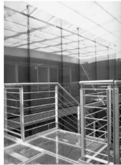
Core atrium of WAT serving as an engine for passive ventilation by a glazed blackwall and as a natural light source by daylight optimization including transparent stairs and galleries
