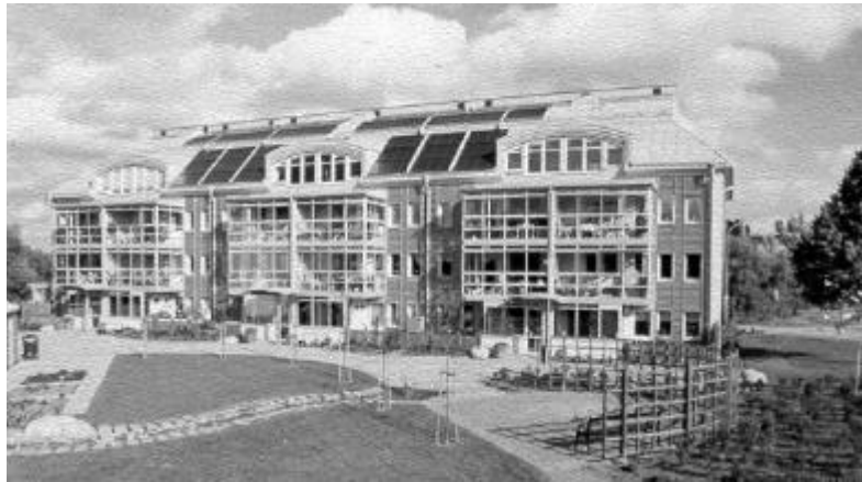
EKOPORTEN in Norrköping, Sweden Multi-unit residential retrofit project addressing overall environmental and energy measures including energy, land and water, material and sewage issues.
