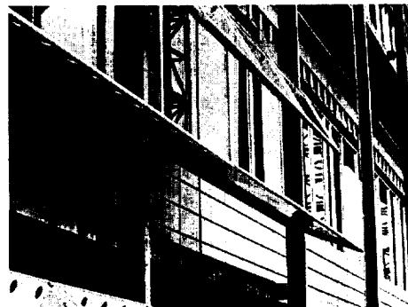
Fig. 2: The sunshading PV system.
