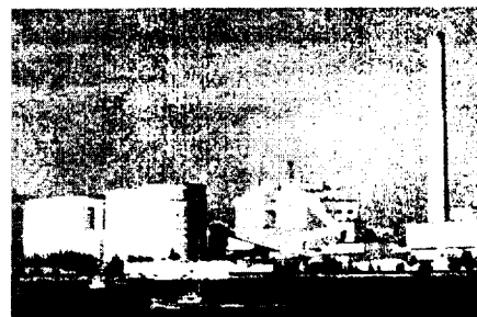
Fig 3 Picture of the coal-fired thermal power plant for calculation
