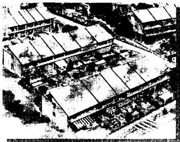
Solar City in Freiburg (Germany) under construction by Disch
