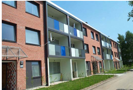
Figure 2 Façade after renovation
