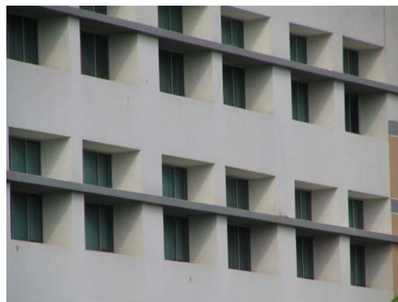
Figure 3: The “Punch Hole” windows provide shading to the windows
