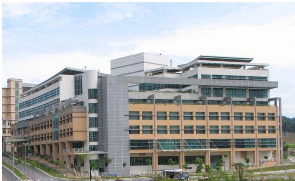
Figure 1: East facade of the LEO Building
