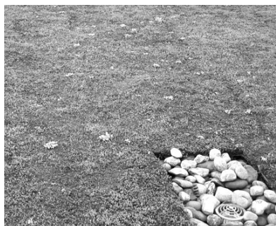
Figure 4 Detail of succulent layer on roof. Protects membrane from ultraviolet degrading.
