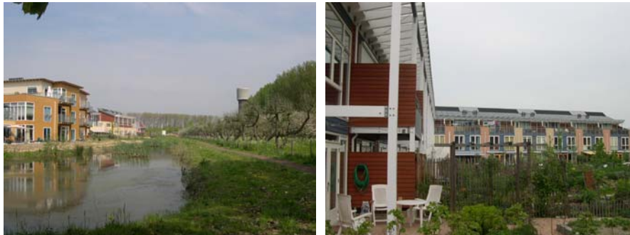
Figure 1 Lanxmeer district with orchard, drinking water extraction area, retention ponds & helophytes (left) and semi-open court yards (right)
