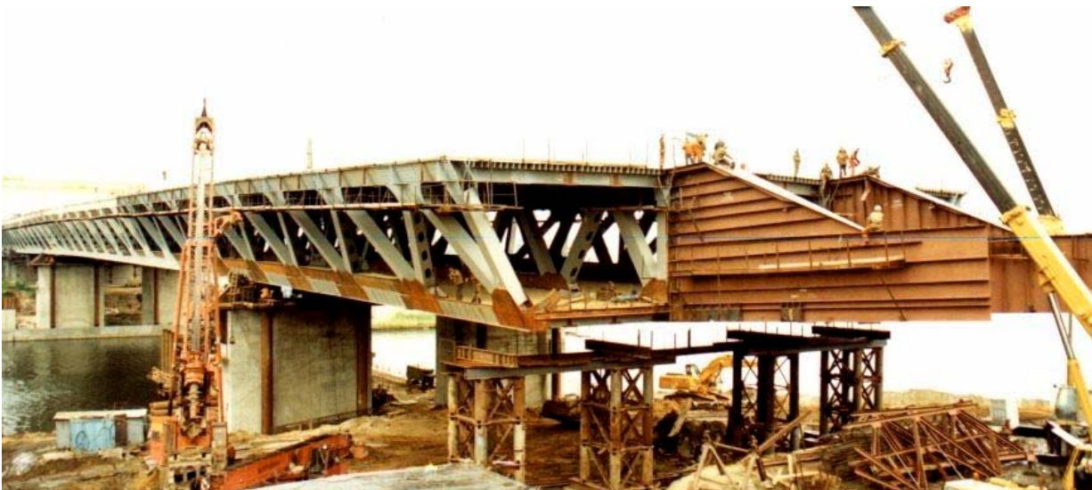
Fig. 1 Position of superstructure before bearing over temporary pier
