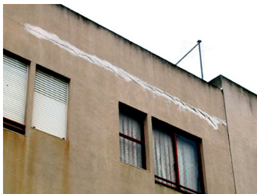
Fig. 1 - Differential cracking in parapet
