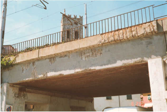
Figure 2 Structure continuing to serve intended function despite active corrosion
