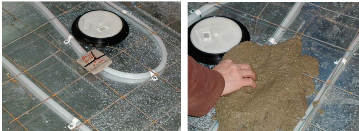
Fig. 3. Pre-cast sensor before casting intermediate floor slab
