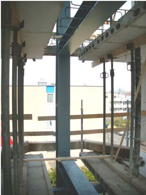
Figure 5. Situation after installation of the steel frame
