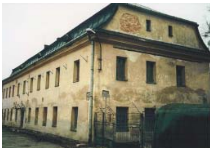
Fig. 1 Historic Building with Crack Formations and Devastated Masonry
