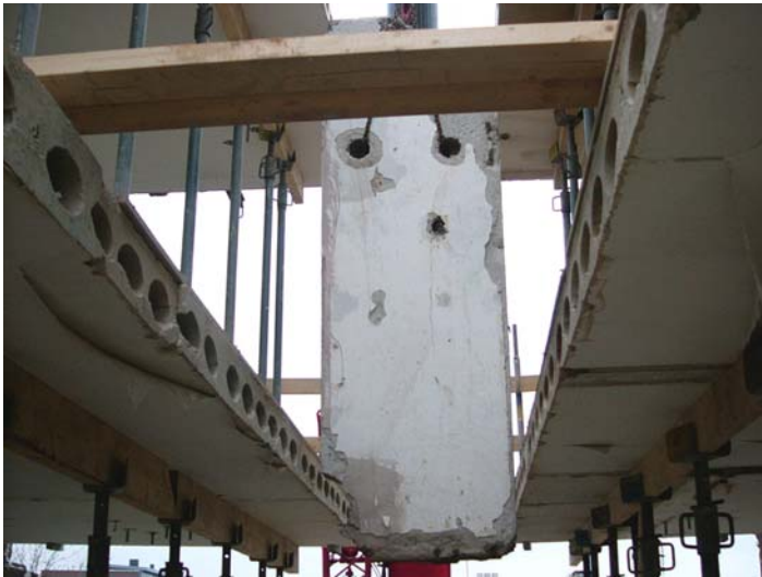
Figure 4. Removal of the bearing wall elements
