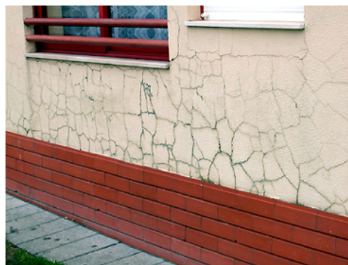
Fig. 2 - Cracking due to render shrinkage
