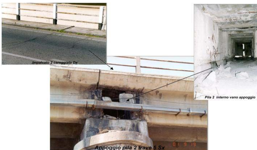
Fig. 3 Degradation of deck near bearings
