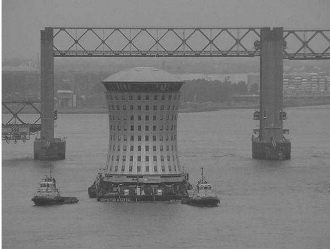
Figure2: A fully factory made office on its way to the foundation.
