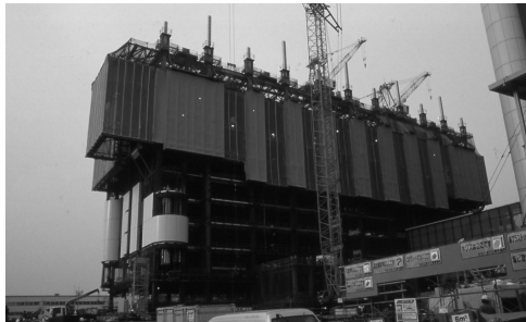
Figure 7 shows an automated construction site in September 2003
