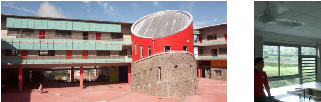
Figure 2 : The three storeys main building with sun shading devices, external corridors facing north and louver windows (right). All the classrooms are cross ventilated with sliding windows, louvers and air fans (left).
