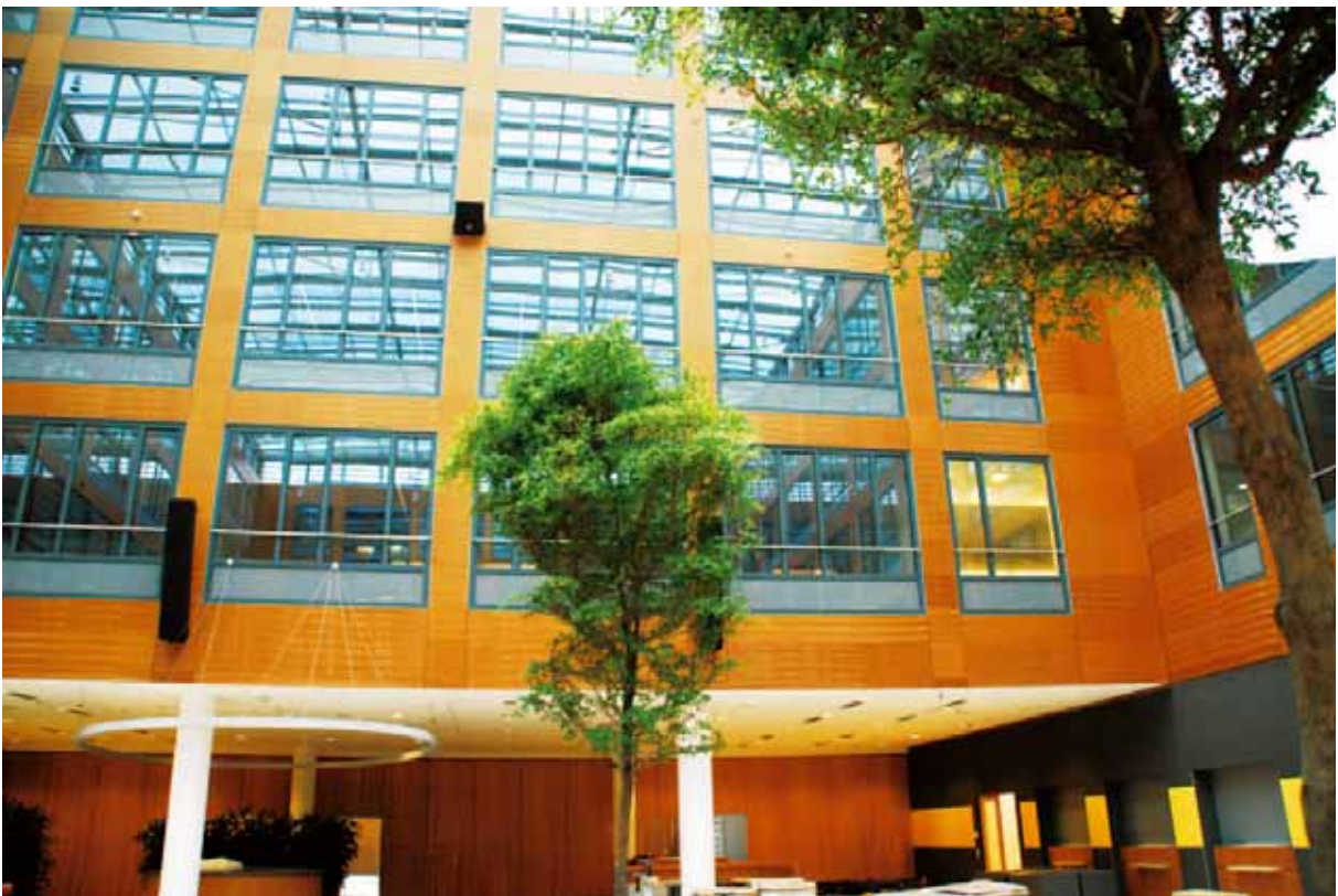
13 Fassade of the customer foyer
