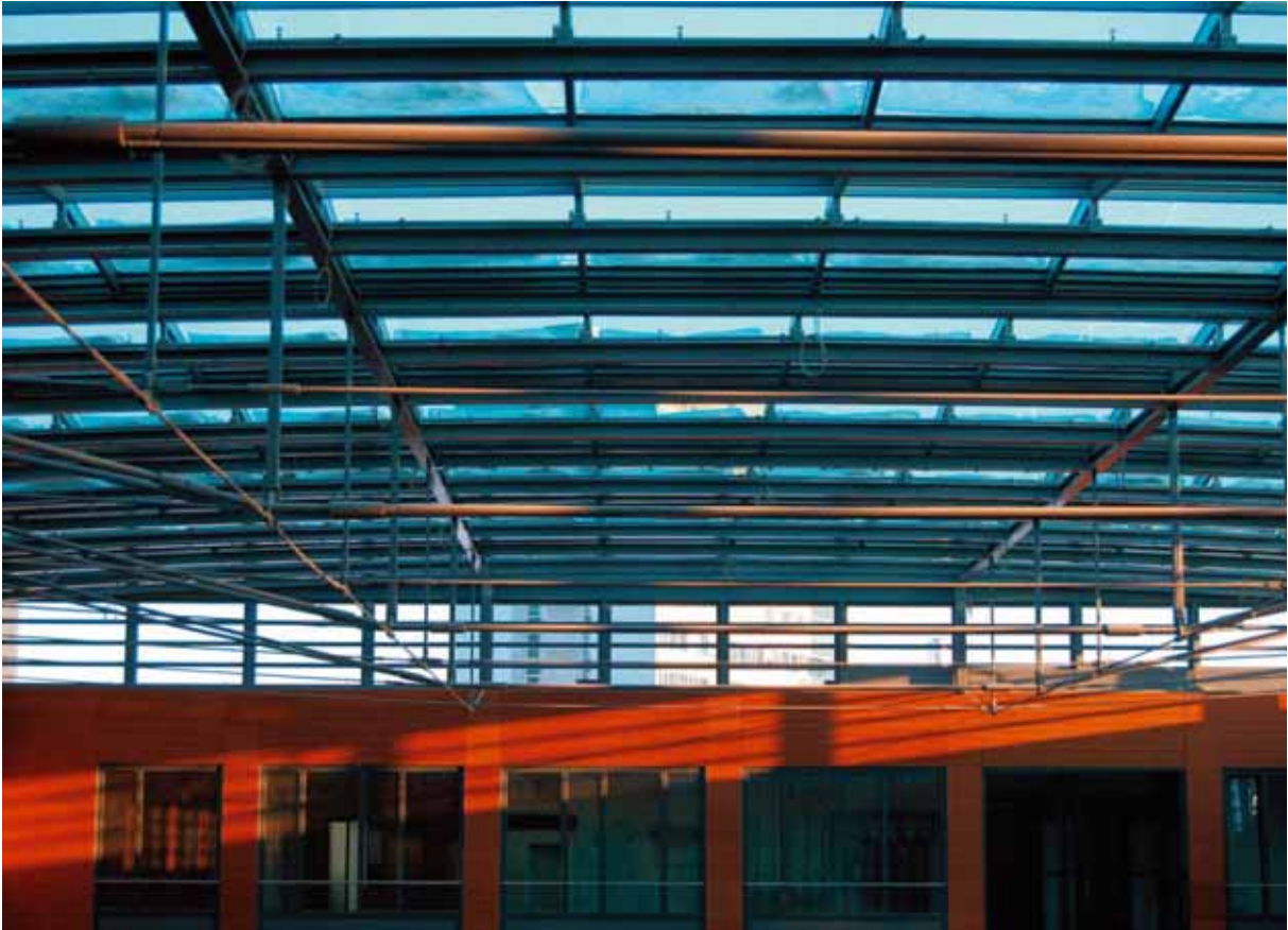
12 Roof structure with ventilation panels
