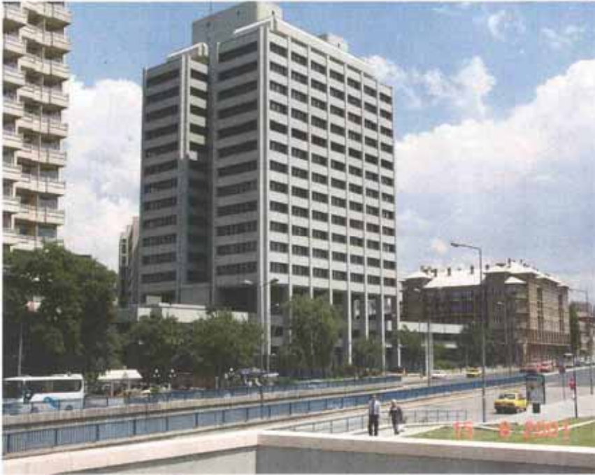
Figure 1. External view of the building.
