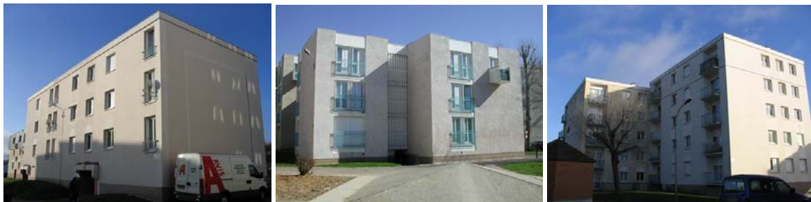
Figure 1 : View of buildings of HR-VENT project.
