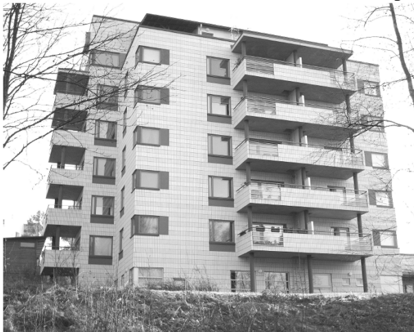
Figure 2. A photo of the simulated apartment building.
