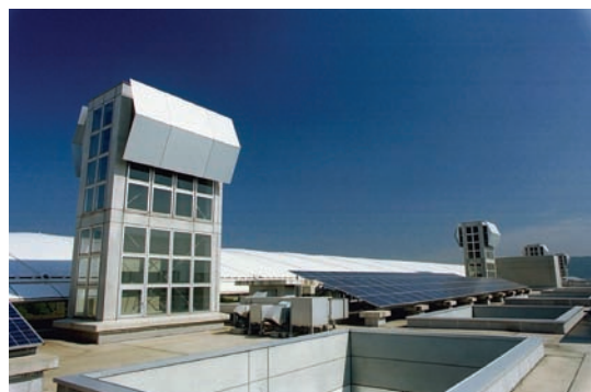
Figure 2. Solar chimney on the roof
