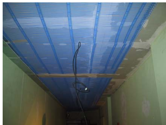
Figure 1. Integrated heating/cooling ceiling system with capillary mats
