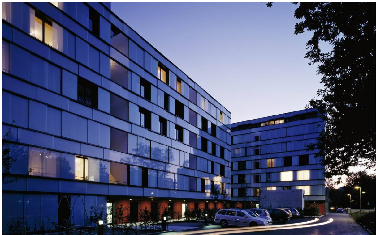
Figure 1. Multiple-family dwelling offering 90 apartments close to Zurich designed to comply with the demands of MINERGIE-P®. (Picture courtesy of Senn BPM, Switzerland)
