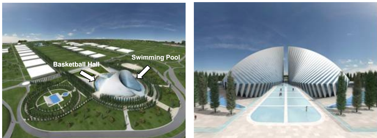
Fig. 1 – “Città dello Sport”, Rome – General view and main building [1]
