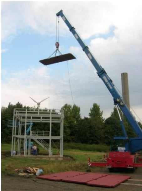
Figure 4: Erection of Modular Research Building
