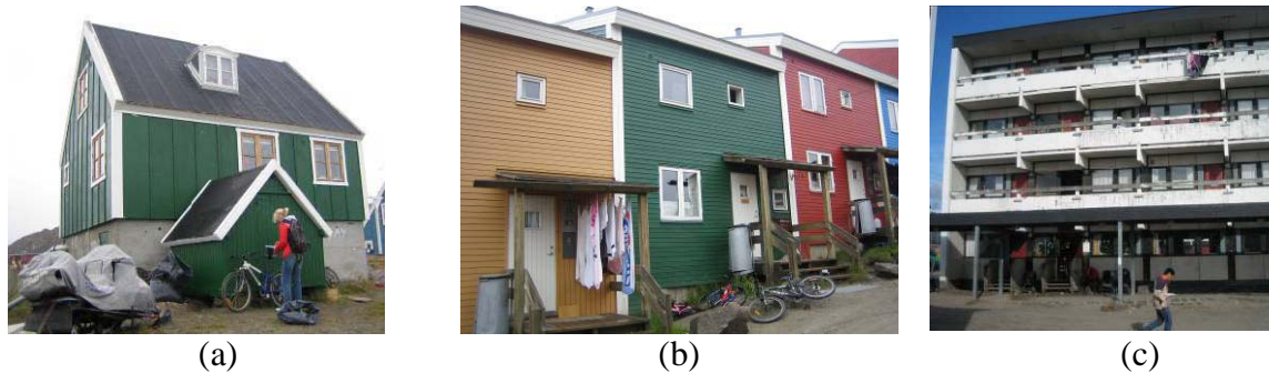
Figure 1. Types of dwelling in Sisimiut. Single family house (a), attached houses (b) and apartments (c).
