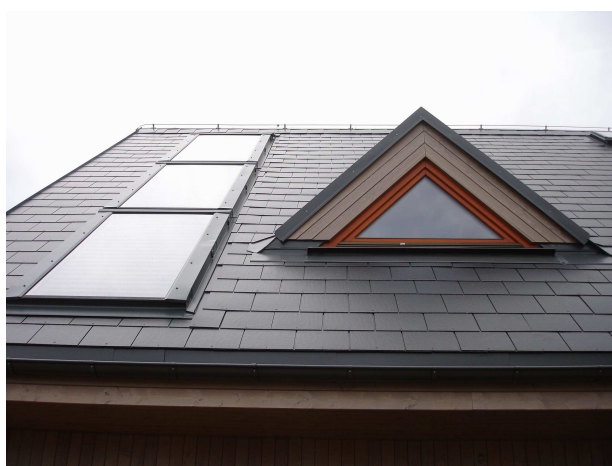
Fig. 2 Roof integrated solar thermal system with carefully designed and performed details
