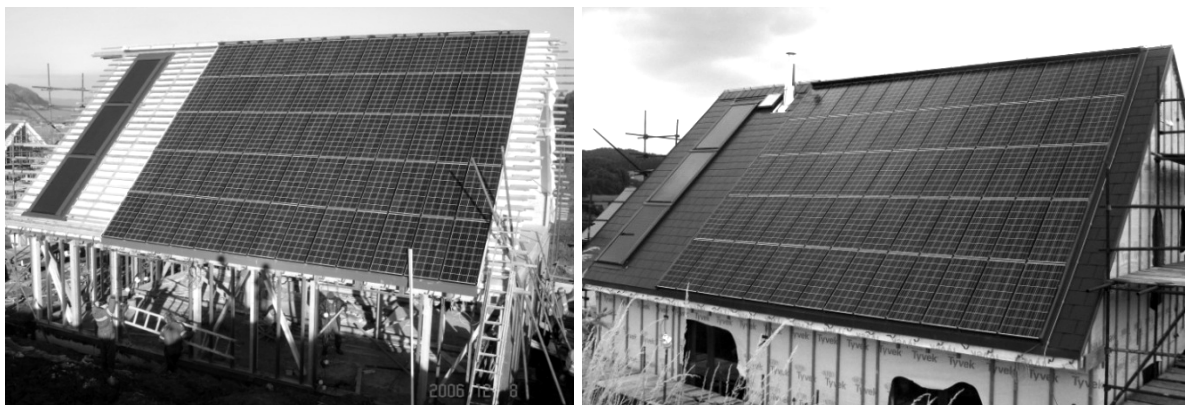
Fig. 6 The pitched roof with 62.9 m 2 large PV array during construction works (left) and completed roof (right)
