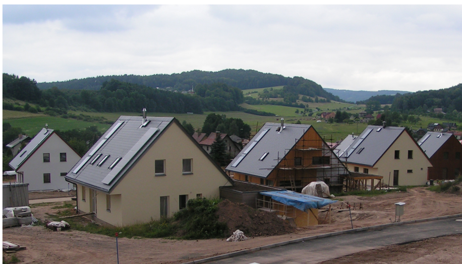
Fig. 1 Part of new residential area in Koberovy – July 2007. All passive houses are equipped with solar thermal collectors, integrated in pitched roofs
