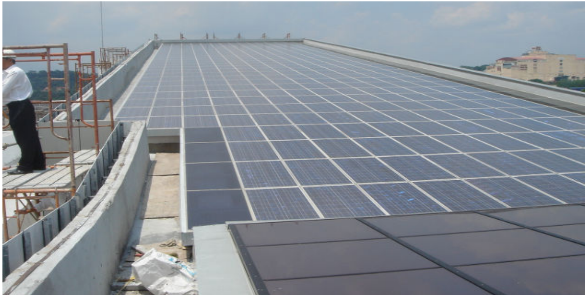
Figure 3 : The larger PV roof, 45 kWp polycrystalline, in the foreground : part of thin film 6 kWp
