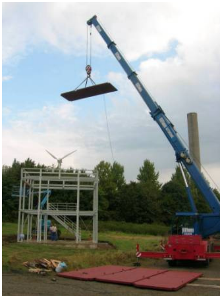
Figure 4: Erection of Modular Research Building
